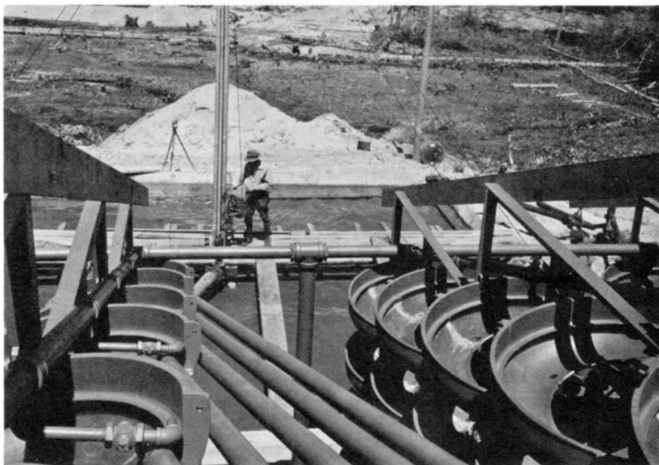
Figure 18. Humphreys spirals during construction of gravity concentration plant by Humphreys Gold Corp. at The Lagoons in 1943.
