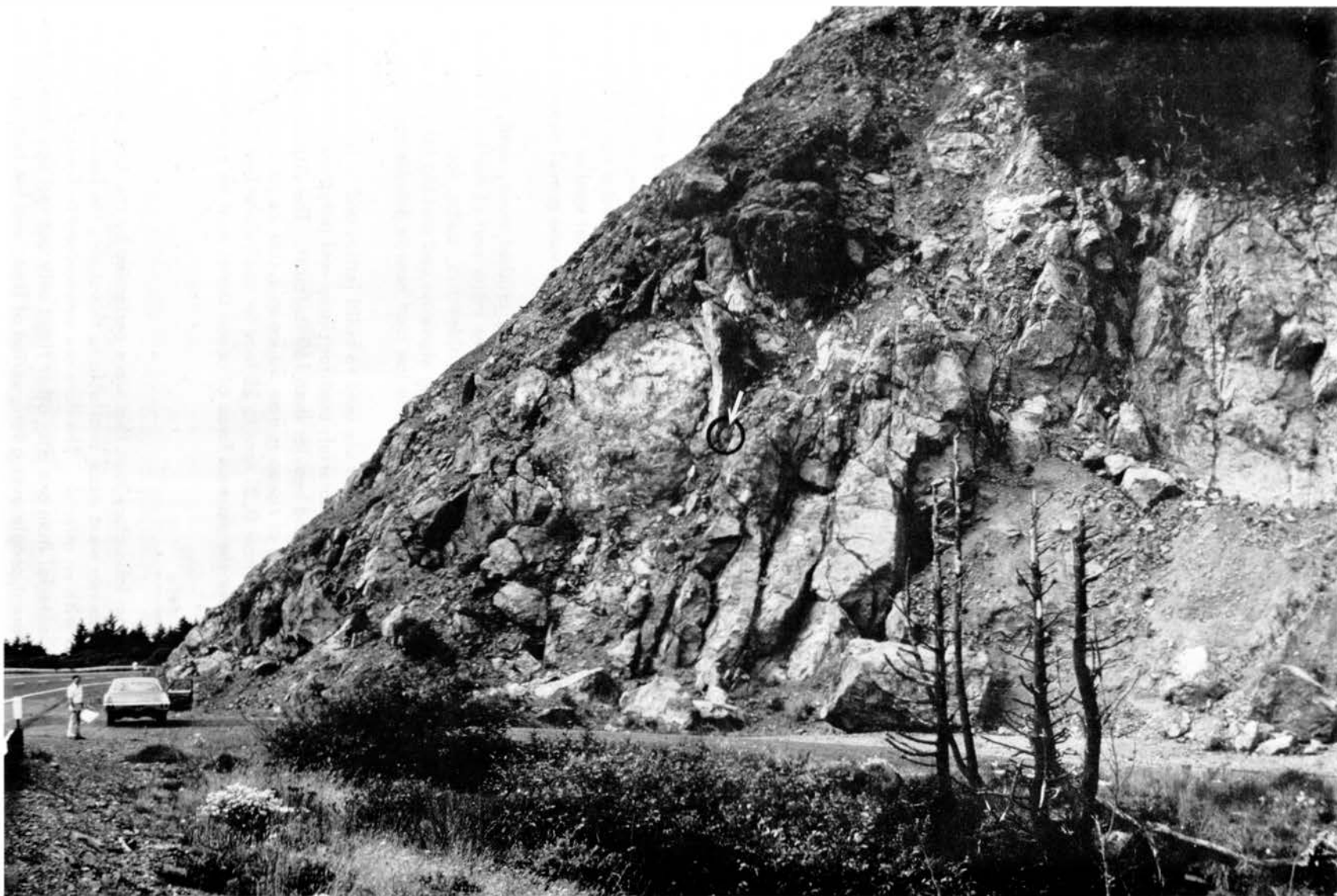
Figure 6. Rock-material site 472, showing unsealed highwall face. Jointing ranges from blocky to massive. Small stone in circle (see arrow) is keystone supporting large stone above.
