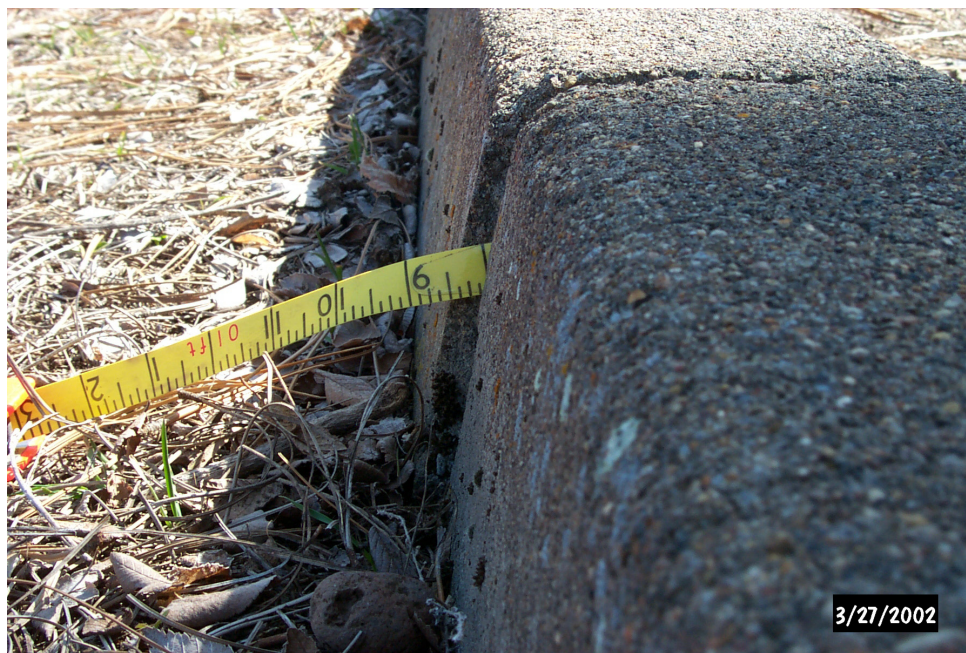
Figure 3.11. Left-lateral offset in curb at parking lot northwest of shear in Figure 3.10. The two shears are connected by a small, northwest-trending notch cut by erosion of apparently sheared soil.
