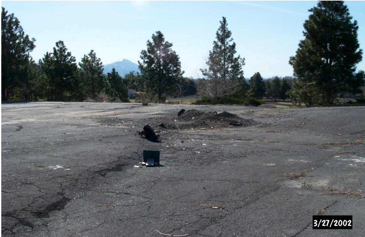
Figure 3.12. Approximately 7-m-wide graben in school parking lot. Backpack is shown for scale.
