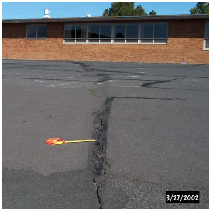
Figure 3.7. Looking northwest at down-to-the-west offset of school parking lot.
