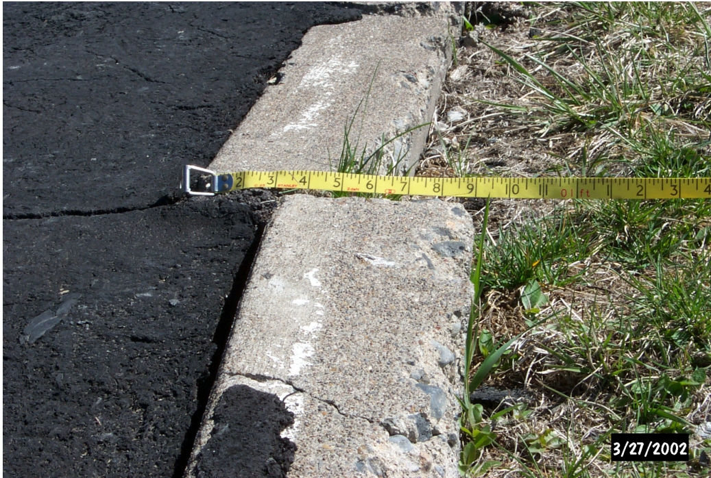
Figure 3.10. Left-lateral shear at north end of running track.
