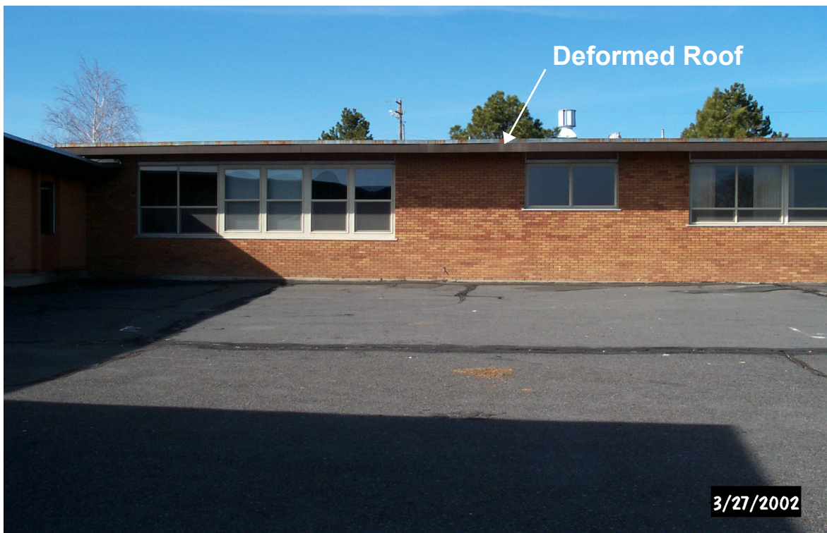
Figure 3.13. Slightly deformed roof line on Ponderosa Junior High School where down-to-the-west (left) ground deformation crosses the building.
