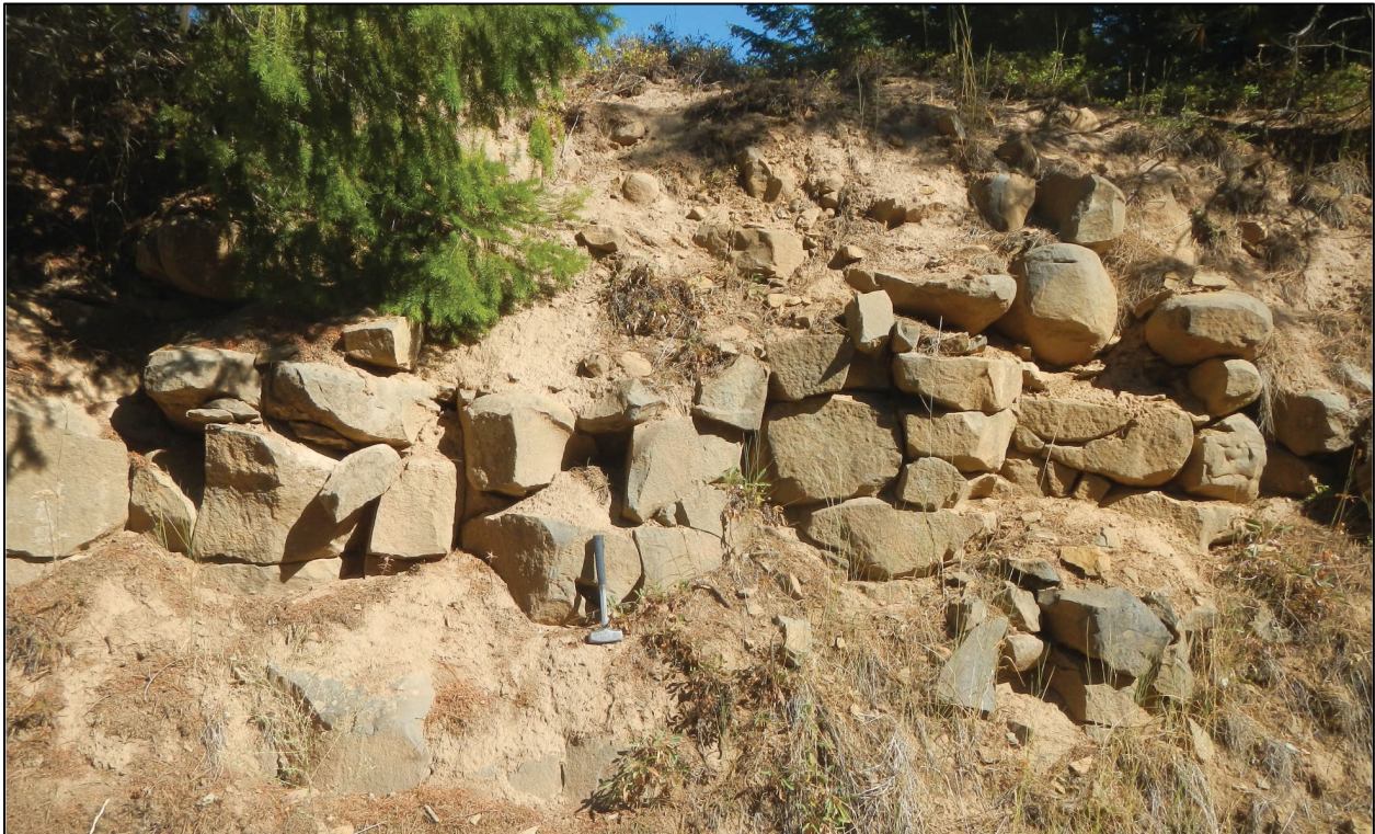
Figure 6-15. Blocky-jointed basaltic andesite of Ward Creek (Qrbw) cropping out along USFS Road 4430 (45.43642, -121.46649). Hammer for scale is 38 cm (15 in) long. View is looking east. Photo credit: Jason McClaughry, 2016.
