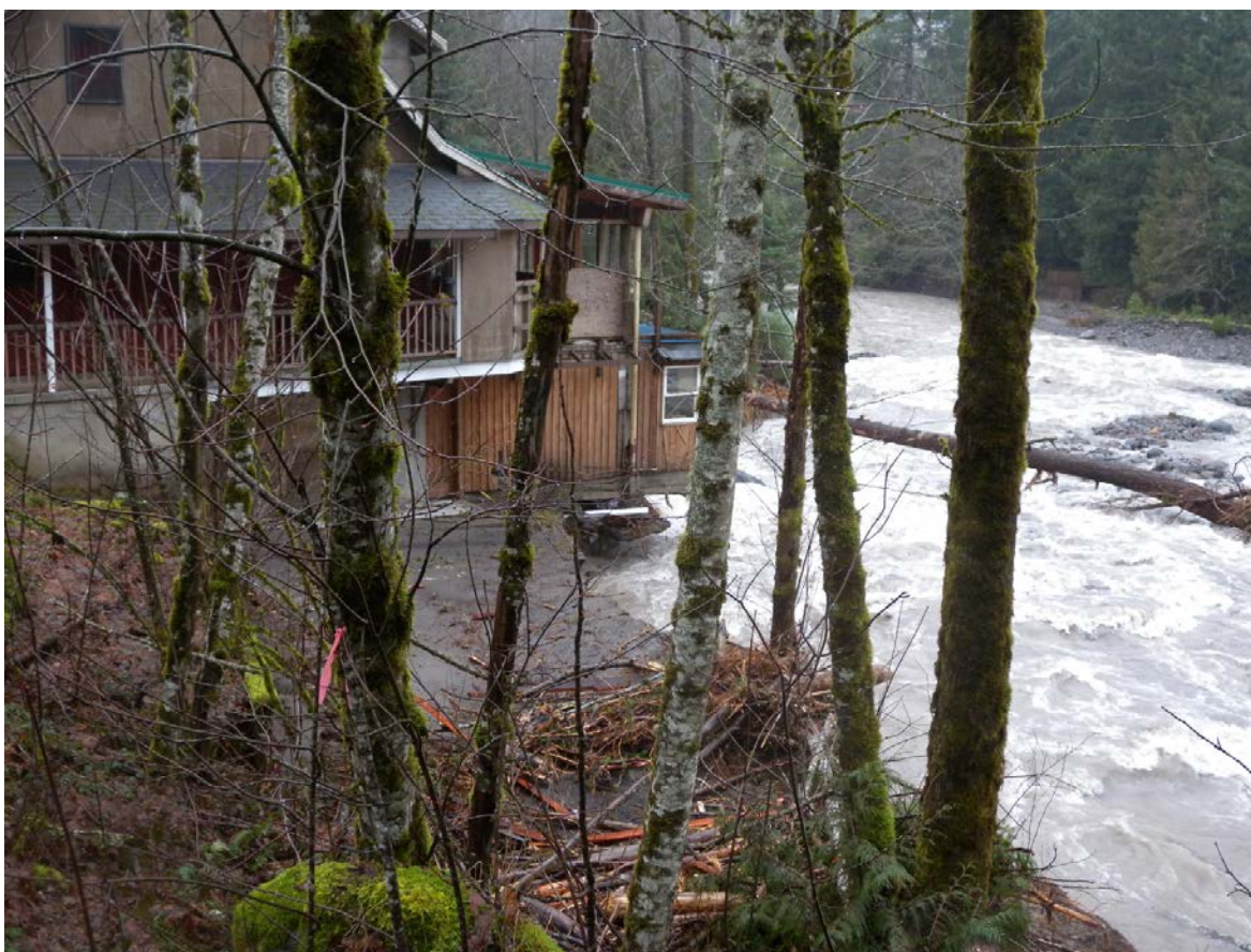
Figure 2-1. Private residence undercut during a flood and channel migration event in January 2011 on the upper Sandy River in Clackamas County, Oregon (photo credit: J. English, DOGAMI, 2011).
