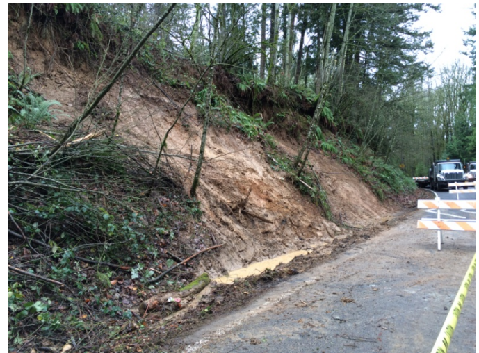
Figure 5. Road cut failure on Southeast Flavel Street after debris cleanup, December 2015.
