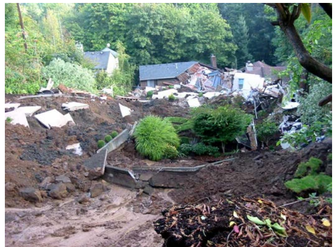
Figure 1. The Burlingame Landslide, in SW Portland, caused estimated losses exceeding $1.5 million in 2008. One house and lot slid down the hill into two other houses. Two houses were complete losses and three houses had moderate to significant damage. The landslide was relatively small at approximately 20 meters wide.
