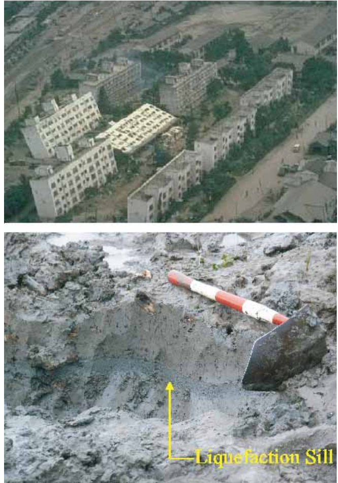
Figure 8. (top) Example of liquefaction induced settlement of apartment buildings, Kawagishicho, Niigata earthquake, Japan, 1964 (Hausler and Sitar, 2001). (bottom) Example of a liquefaction sill at Hunting Island along the Columbia River. The sill most likely is a result of the last Cascadia Subduction Zone earthquake (in 1700 AD).
