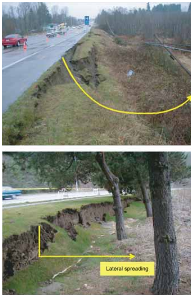
Figure 9. (top) Road prism rotational type landslide and (bottom) lateral spread landslide along the shoreline of Capitol Lake Olympia, Washington, caused by the 2001 magnitude 6.8 Nisqually earthquake (Nisqually Earthquake Information Clearinghouse, 2001).
