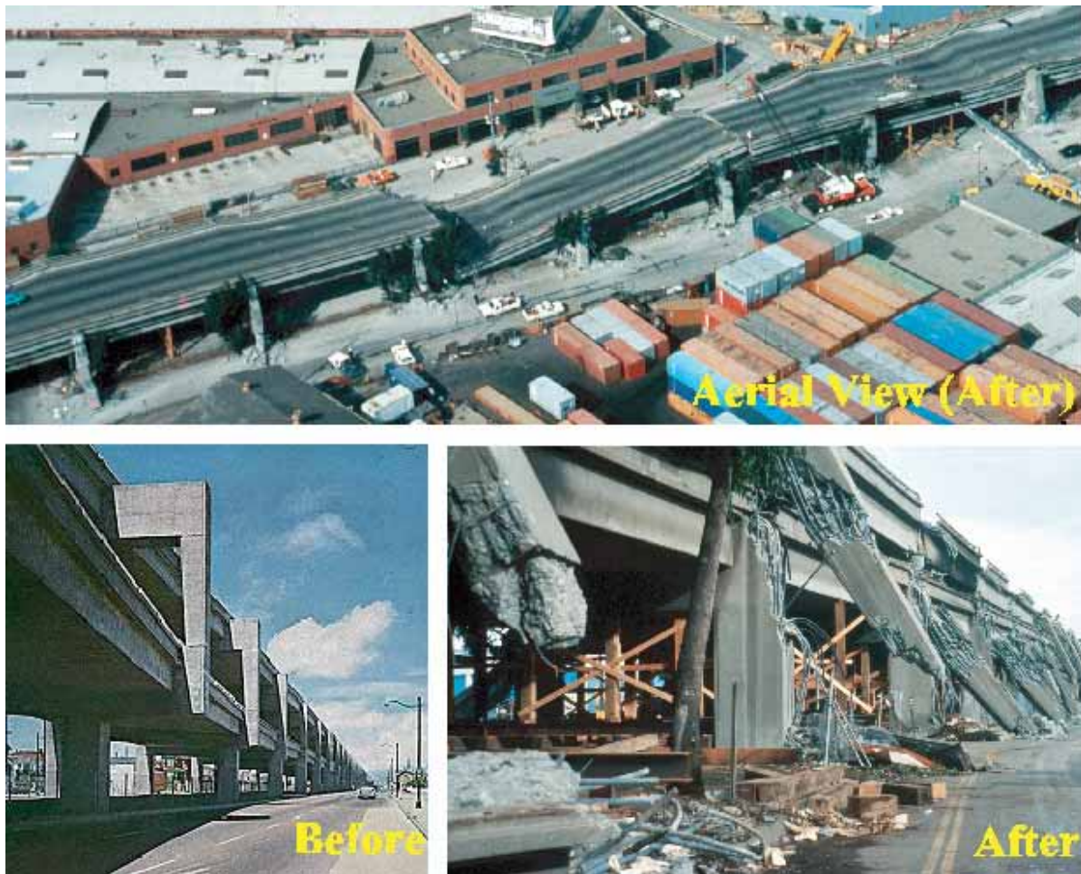
Figure 7. Example of damage to the Cypress viaduct of Interstate 880 caused by ground-shaking amplification during the October 17, 1989, Loma Prieta, California, earthquake (top: Nakata and Peterson, 1990) (bottom: Windmiller, 2000).
