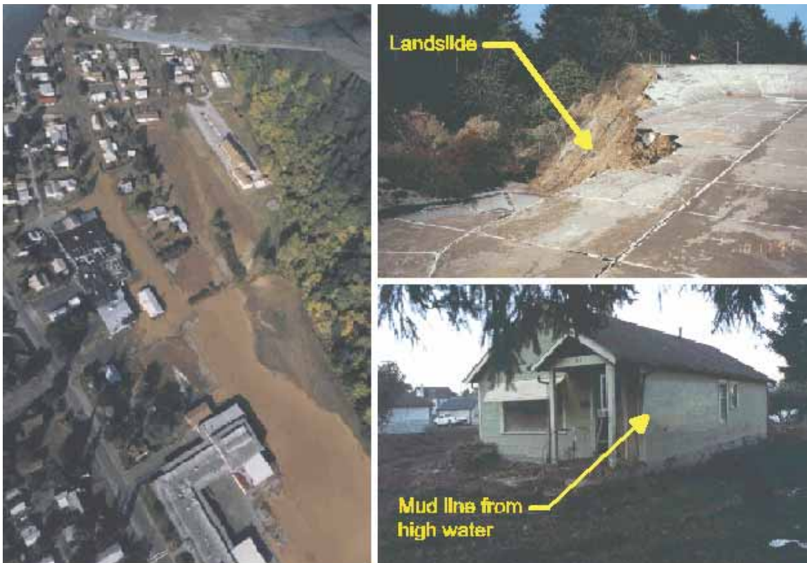
Figure 15. Seminary Hill Reservoir dam failure caused by a landslide. Portions of the City of Centralia, Washington, were inundated. (Washington State Department of Ecology, Water Resources, 1991).
