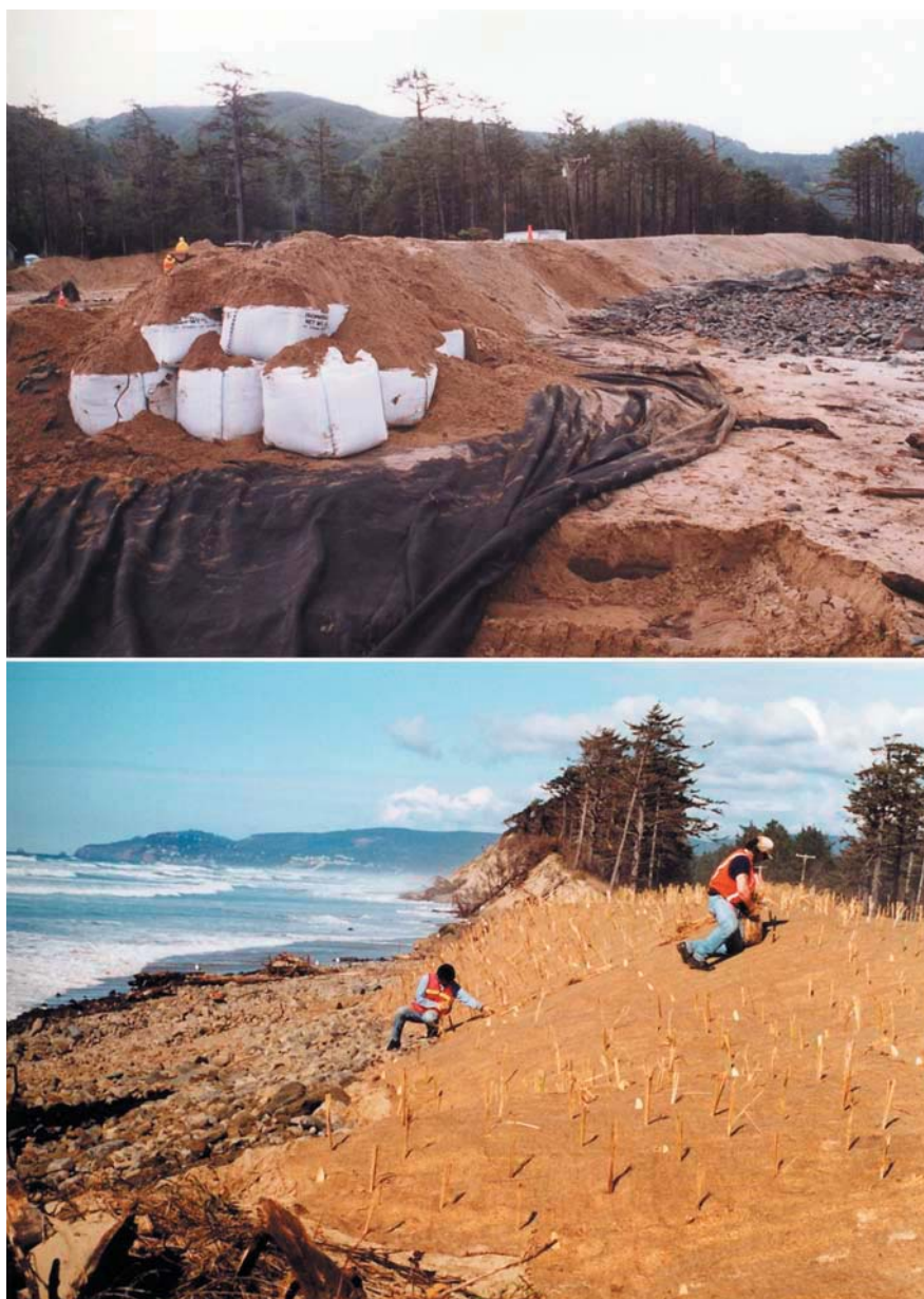
Figure 18. The completed cobble revetment in July 2001, backed by a line of reconstructed artificial dunes containing a core of sand-filled geotextile bags. Recent storms have deposited drift logs atop the dunes, while sand carried by summer winds has also begun to accumulate and cover the cobble berm (Jonathan Allan photo).
