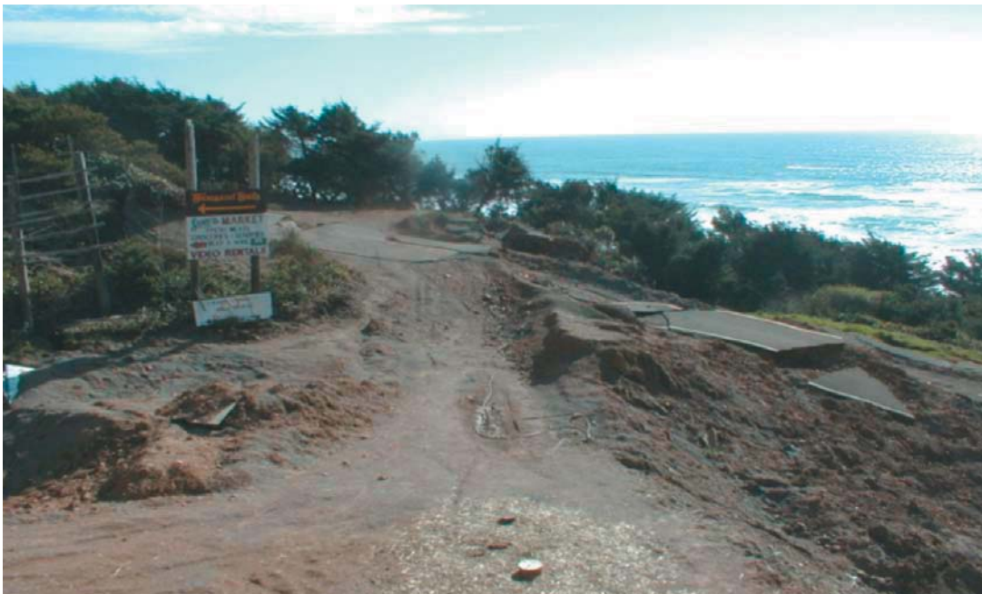
Figure 15 Complex oceanfront landslide on Three Capes Loop Road between Pacific City and Sand Lake.
