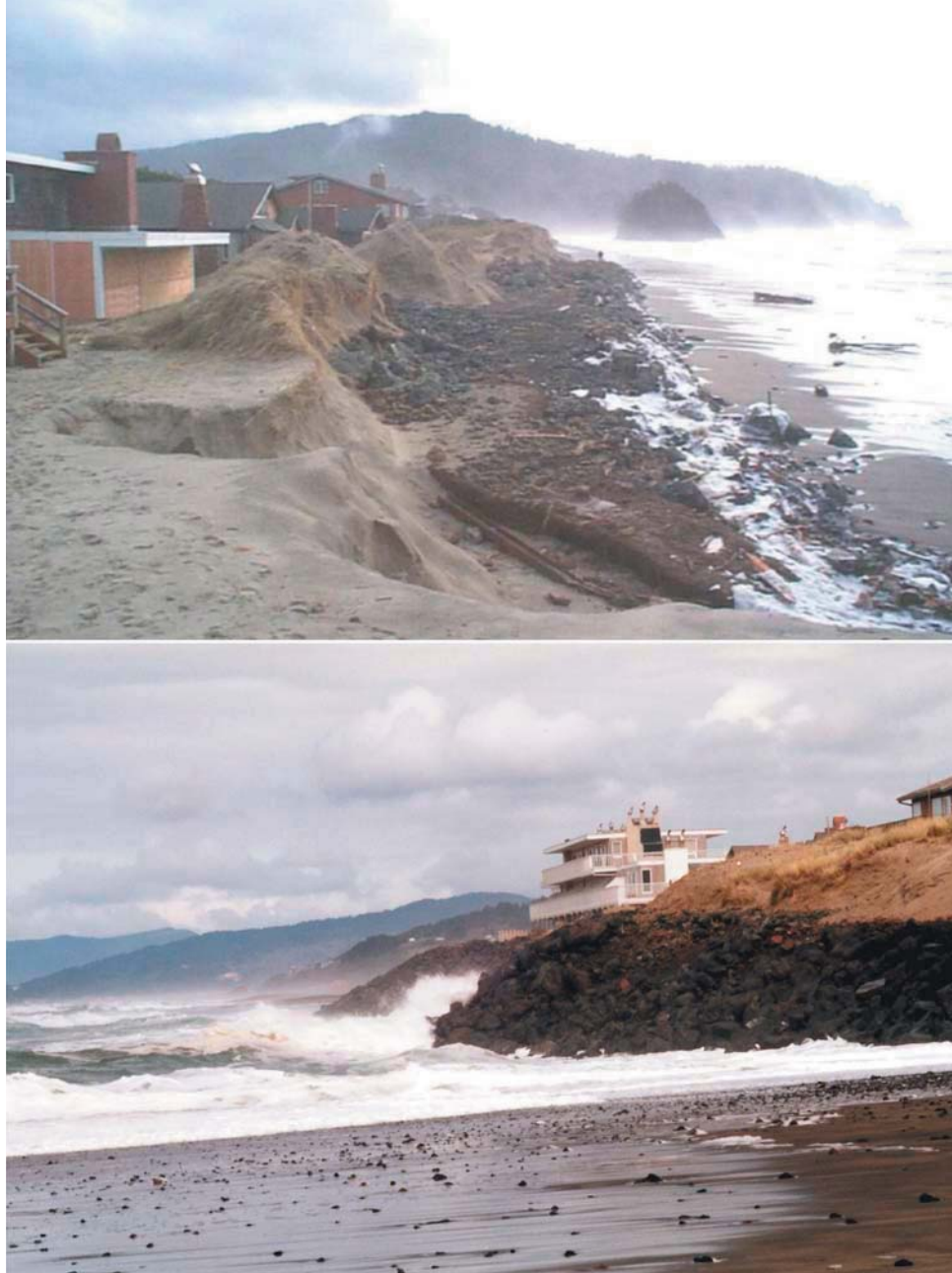
Figure 8. (upper): Emergency riprap in place along Neskowin shoreline, spring 1999 (Oregon Parks and Recreation Department photo). (lower): Final riprap structures at Neskowin in winter 2001 following regular permit process. Note that the structure has blocked lateral access along the beach at low tide due to enhanced erosion of the beach in front of the structure caused by the presence of a rip embayment and from wave reflection off the structures (Paul D. Komar photo).
