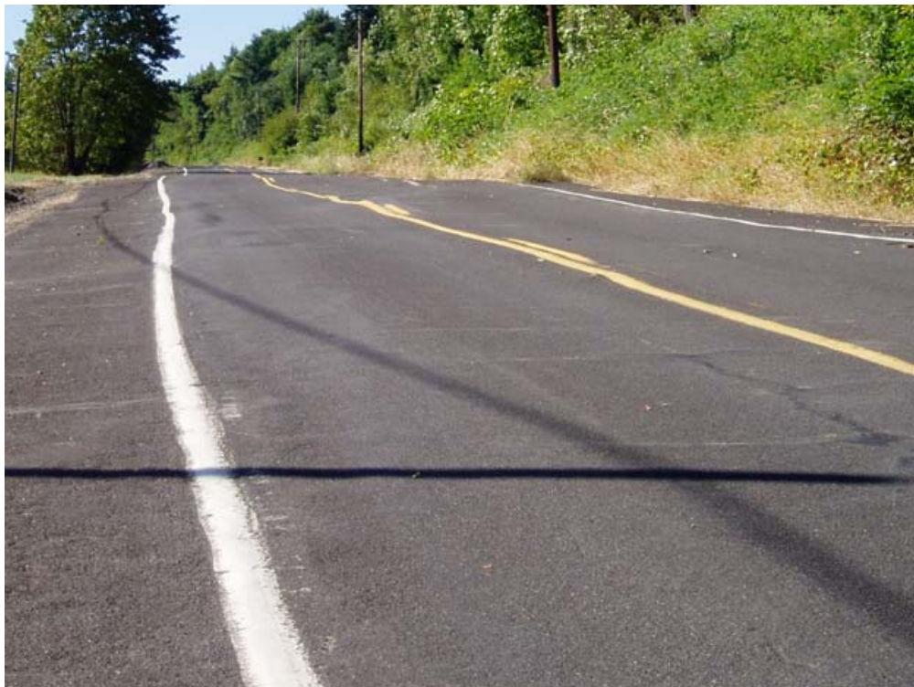
Figure 6. Active landslide. Buckled pavement along Rocky Point Road just off the eastern edge of the Dixie Mountain quadrangle where the active toe of a bedrock landslide (unit Qlb1) in the Dutch Creek complex (unit Plld) is moving. View south from station PDX-962 (NAD 83 UTM coordinates 509,766 m E, 5,062,127 m N).
