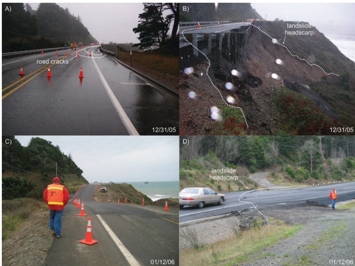
Figure 2. A) The Rocky Creek landslide on December 31, 2005, with surface cracks extending across the western lane of U.S. Highway 101; B) the western lane of the highway is undermined due to a slump/block failure (note the head scarp running seaward near the top-right center of the photo); C) the main slump on January 12, 2006, which caused Highway 101 to drop by approximately 6 m (20 ft); D) surface cracking on January 12, 2006, some 230 m (760 ft) north of the main slump/block failure across Rocky Creek, indicating other movements in the area.
