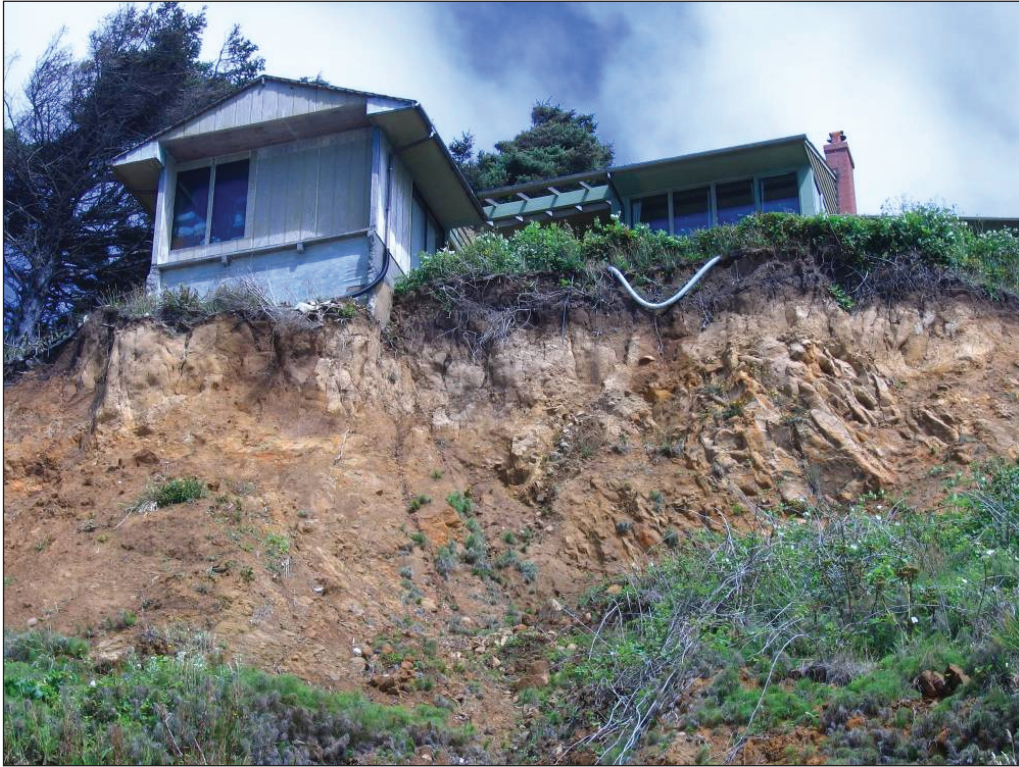
Figure 33. Chronic erosion and land sliding along Cove Beach has required many homeowners to modify or move houses away from retreating sea cliffs. Large, jointed sandstone blocks surrounded by sand and silt are inferred to reflect late Pleistocene rock avalanche deposits.
