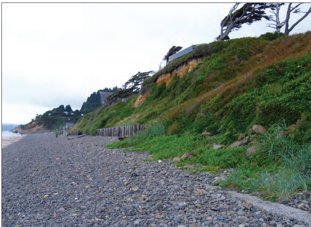
Figure 29. Wood pilings form a rudimentary sea wall (middle distance) along Arch Cape. Bluffs 20 to 30 ft high in late Pleistocene coastal terrace deposits expose dense, cemented gravels (above sea wall).
