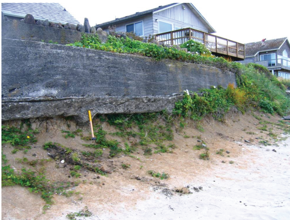
Figure 18. Example of a seawall in Cannon Beach that has been undermined by wave erosion.
