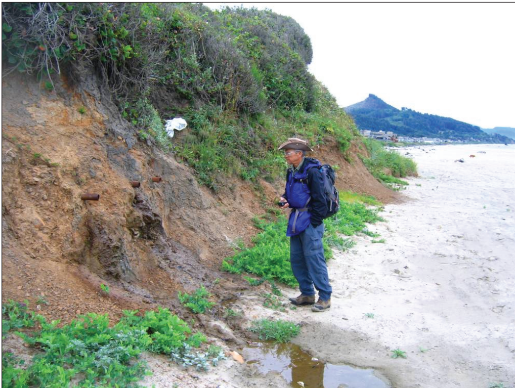
Figure 21. Horizontal drains exposed at the toe of the S-Curves landslide consist of 150- to 300-ft-long, 1.5-in slotted PVC pipe. The drains carry away ground water for the purpose of lowering the water table and potentially stabilizing the S-Curves landslide in Cannon Beach (Horning, 2004).
