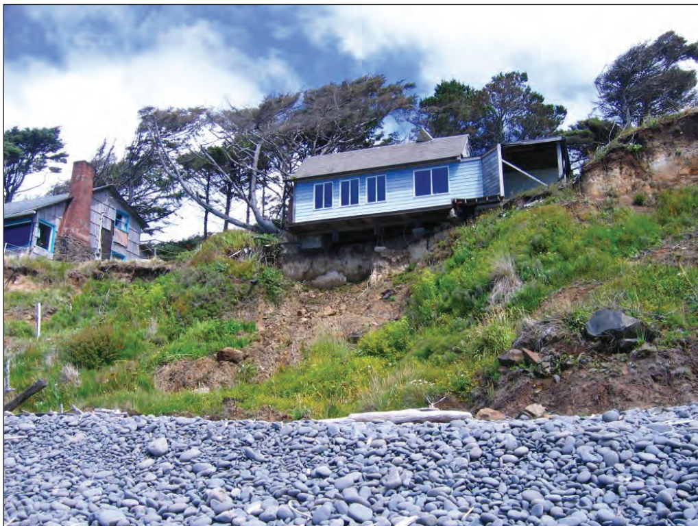
Figure 34. House undermined by bluff collapse due to wave erosion, southern part of Cove Beach.
