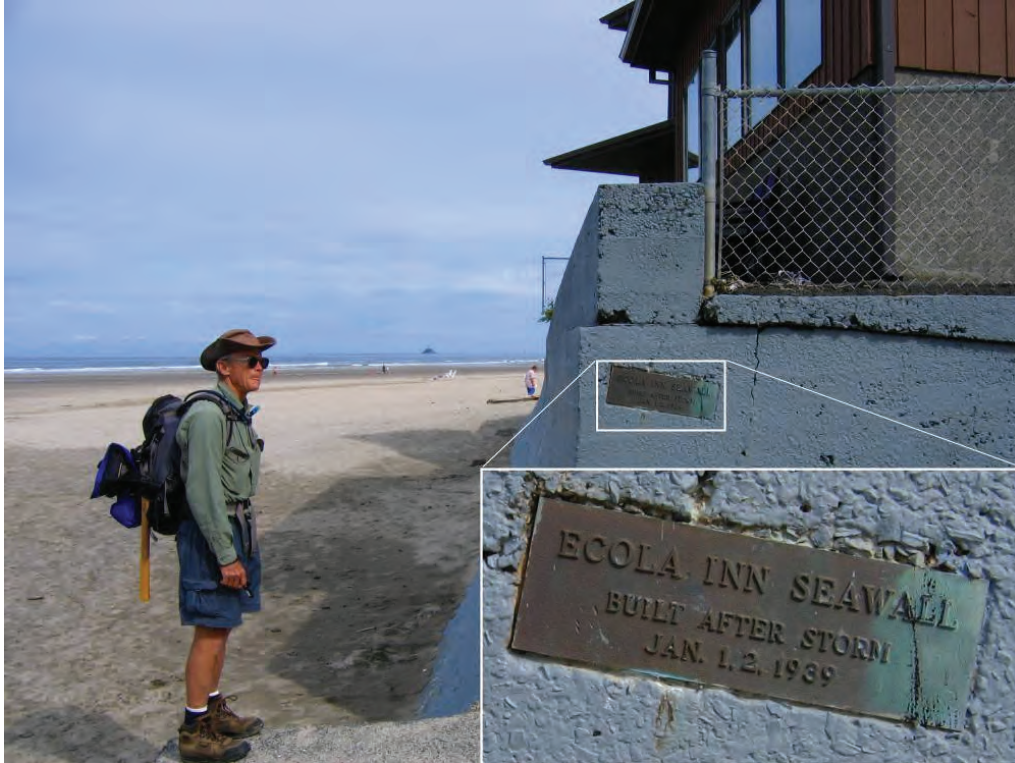
Figure 17. Forty-eight-percent of the shoreline of Cannon Beach is armored with sea walls or riprap to mitigate coastal erosion. This seawall was built after a severe winter storm in January 1939.
