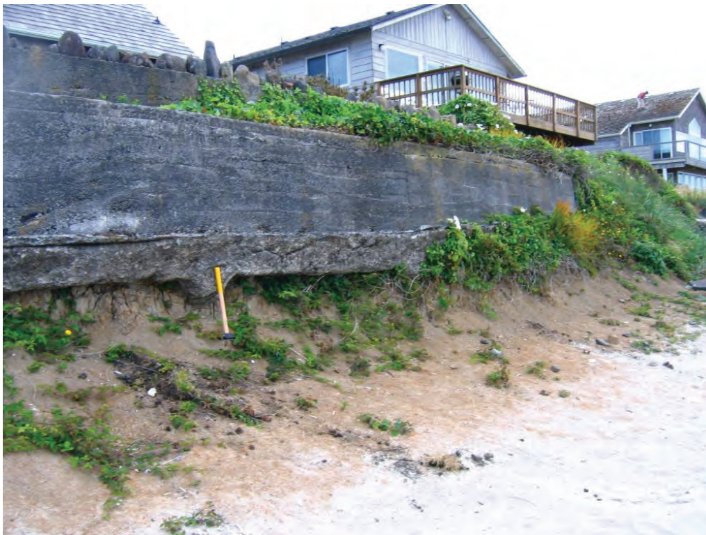
Figure 18. Example of a seawall in Cannon Beach that has been undermined by wave erosion.
