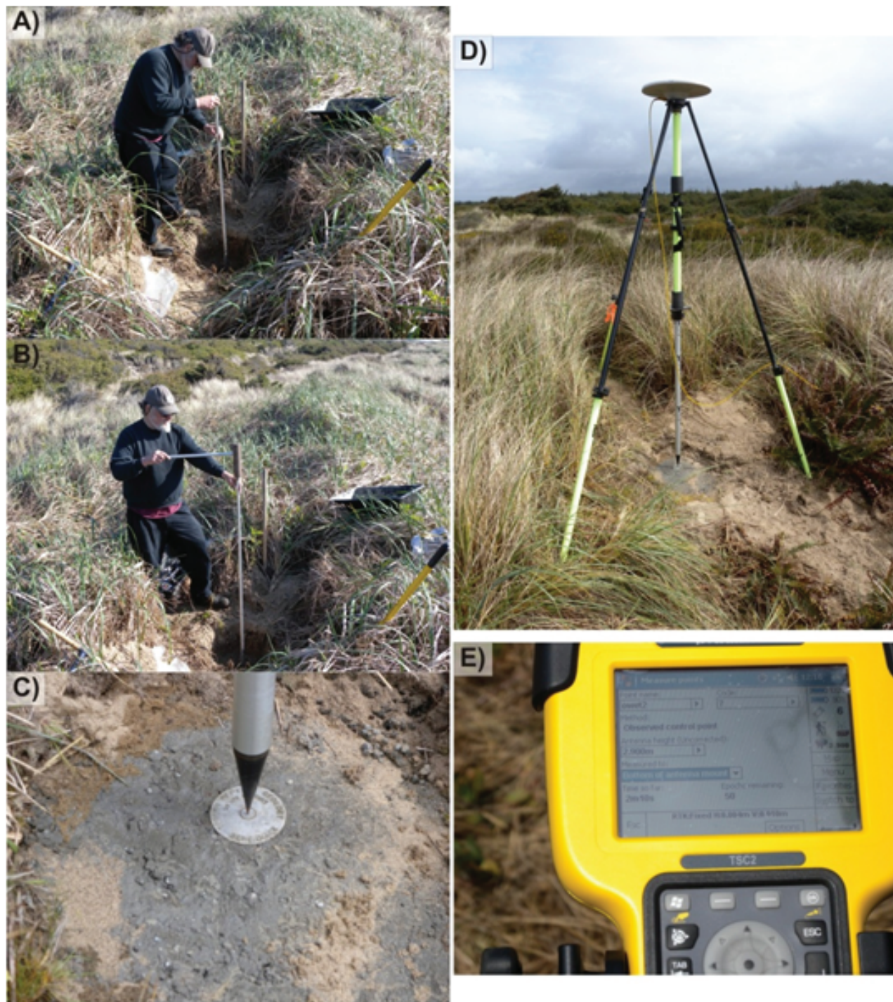
Figure 3. A) Installation of survey benchmarks involved digging a 1 m (3 ft) deep (10-inch diameter) hole, B) hammering sectional aluminum rods to depths of 4–8 m (12–24 ft), then C) capping the rods and concreting in place. D) GPS observation of the OWET 1 survey monument. E) Site calibration is performed on the OWET 2 benchmark using the Trimble TSC2 controller.
