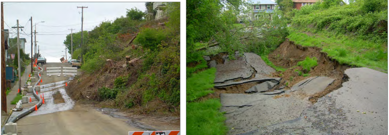
Figure 20. Photos of the First and Commercial Street landslide near the toe along Bond Street (left) and the head scarp along First Street (right).
