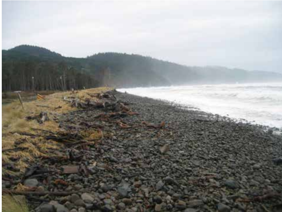
Figure 2-16. A dynamic revetment “cobble beach” constructed at Cape Lookout State Park. The cobble beach is backed by an artificial dune, which is overtopped periodically during major storms. (Photo: J. Allan, DOGAMI, 2008)
