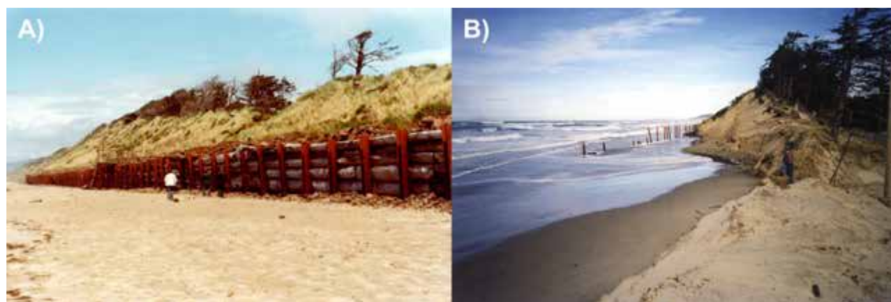
Figure 2-15. A) Wooden bulkhead constructed at Cape Lookout State Park (photo: Oregon Parks and Recreation Department, June 1978); B) The same area in February 1998. (Photo: P. Komar)
