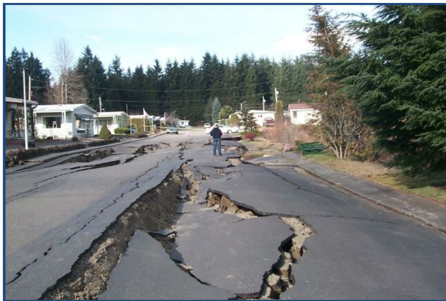
Figure 1-4. Damaged road due to liquefaction-induced lateral spreading, 2001 Nisqually, Washington magnitude 6.8 earthquake. Photographic credit: DOGAMI archives.
