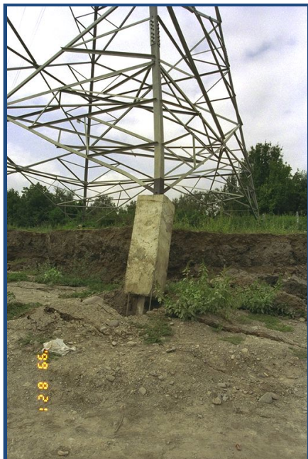
Figure 1-3. Example of ground failure underneath a transmission tower, 1999 İzmit magnitude 7.6 earthquake (Turkey). Photographic credit: University of California, Irvine, Consortium of Universities for Research in Earthquake Engineering archives.
