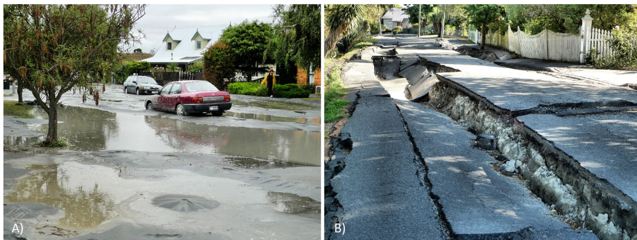
Figure 2-1. Water-saturated sand can turn to quicksand during strong shaking, forming sand boils, ponding, and sunken roads. In these examples, (left) extensive liquefaction occurred along River Road in Christchurch, New Zealand following the February 2011 earthquake, while (right) effects from lateral spreading along numerous Christchurch roads constructed next to waterways resulted in major failures to road infrastructure as roads slumped toward river channels. During a Cascadia subduction zone event, such processes could compromise tsunami evacuation routes, as well as the time and speed to safety in areas prone to liquefaction. (Photo credits: Martin Luff, licensed under CC BY-SA 2.0)
