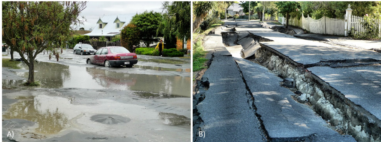
Figure 2-1. Photos of liquefaction and lateral spreading in Christchurch, New Zealand following the February 2011 earthquake. Water-saturated sand can turn to quicksand during strong shaking, forming sand boils, ponding, and sunken roads. (A) Extensive liquefaction along River Road. (B) Lateral spreading along one of many roads constructed next to waterways. During a CSZ event, such processes could compromise tsunami evacuation routes, as well as the time and speed to safety in areas prone to liquefaction. (Photo credits: Martin Luff, licensed under CC BY-SA 2.0)
