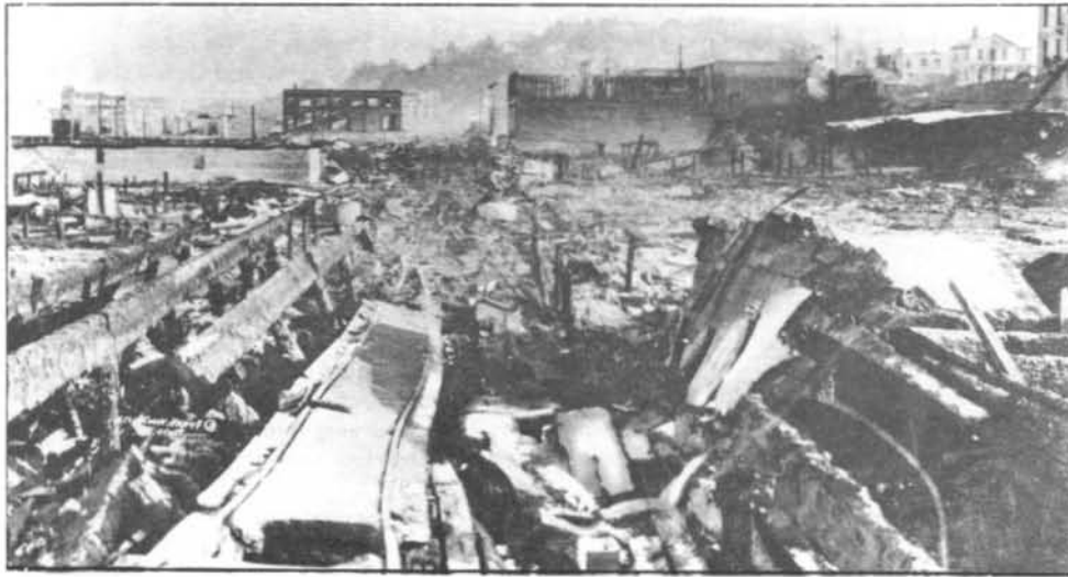
Figure 5. Astoria looking west, after the fire of 1922. To the extreme upper left is the old St. Mary's building. In front of the building notice the broken wooden street and the burned piles on which it was built. In the middle distance is the Court House, which appears in figure 6. (Photo by Frank Woodfield, courtesy, Oregon Historical Society)
