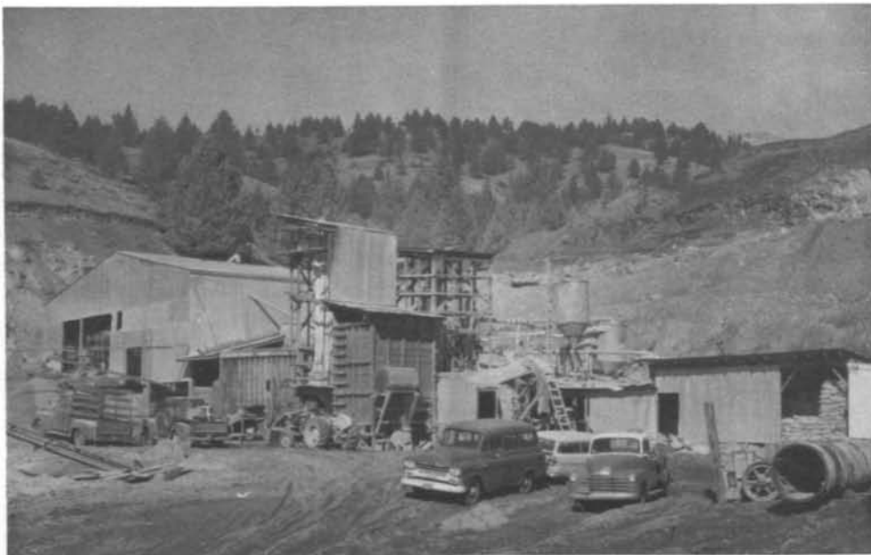
Figure 1. Coast Asbestos Co.'s pilot mill in Grant County, Oregon, 1962. Primary crushing and drying facilities are housed in large building on left side of picture and the storage shed for sacked fiber is on the extreme right. Supplemental processing and sacking facilities occupy intermediate building space. A portion of one of the pits from which ore is taken is shown in rear.
