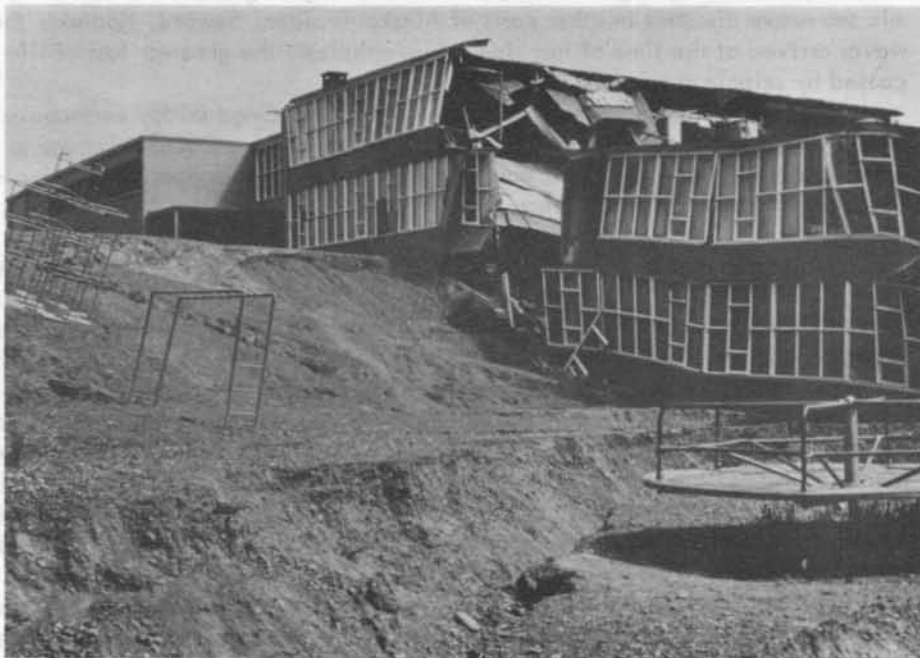
West Anchorage High School with once-level playground destroyed by landslide, Anchorage, Alaska. Photograph by Donald R. Herrick.
