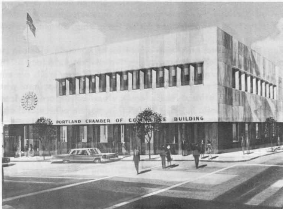
Portland Chamber of Commerce Bldg., 824 S.W. 5th Ave. (bottom). A complete renovation of the old building uses Cold Springs granite facings from Minnesota, and white concrete with white exposed aggregate pre-cast panels. (Photo by Ackroyd)
