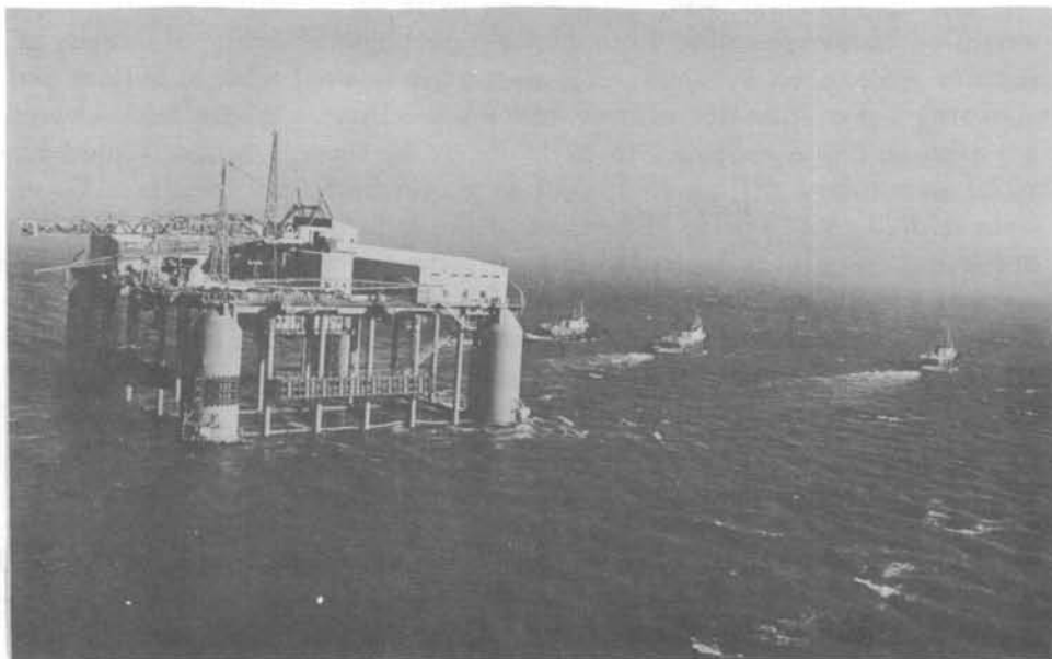
Figure 2. Blue Water II, a huge floating platform owned by the Santa Fe Drilling Co., is shown being towed to one of the drilling sites off the Oregon coast. The equipment was used to drill six of the seven deep holes off the Northwest coast during 1965-1966. (Photograph courtesy Crowley Launch & Tugboat Co., San Francisco, Cal.)
