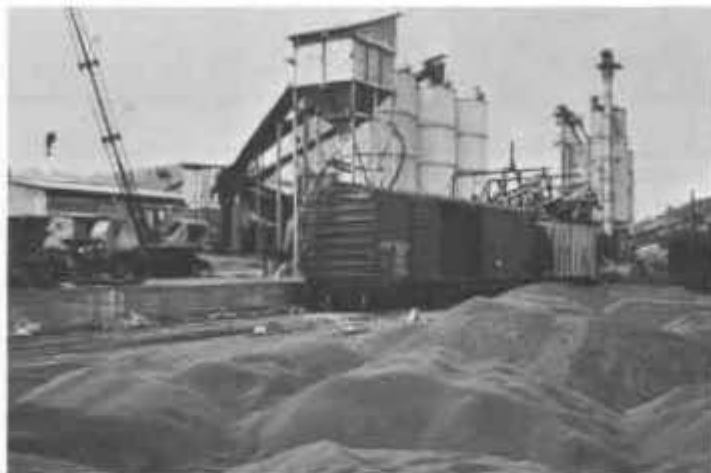
Figure 1. A general view of the "Green Diamond" plant at Riddle, Oregon 1971. The large storage tanks with their associated conveyors are the bulk loading facility; rotary dryer and screening circuits are behind the storage tanks. The bagging facility is at the left. Piles of granulated slag in the foreground.
