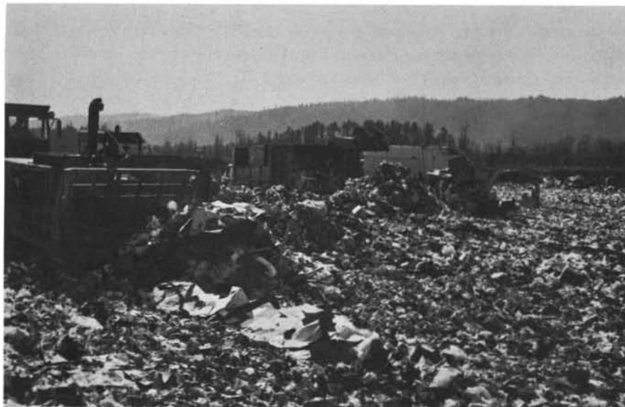
The Swift Blvd. fill has two working faces; one for commercial users and the other for private use. An average of 1000 tons of refuse is dumped each day at this site.
