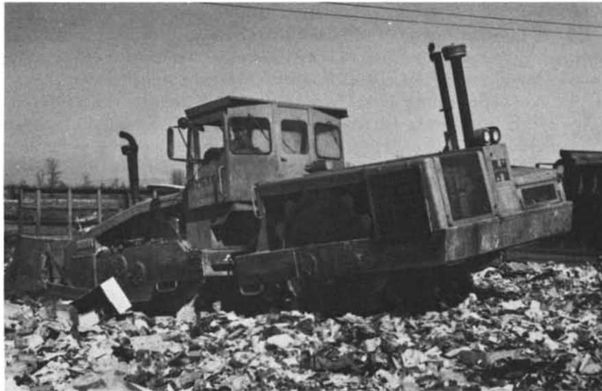
Compacter working on fill at the Swift Blvd. site. After 10 or 12 inches of refuse is spread it is compressed with the compacter. Ten-foot layers of compressed fill are alternated with 2-foot layers of soil.
