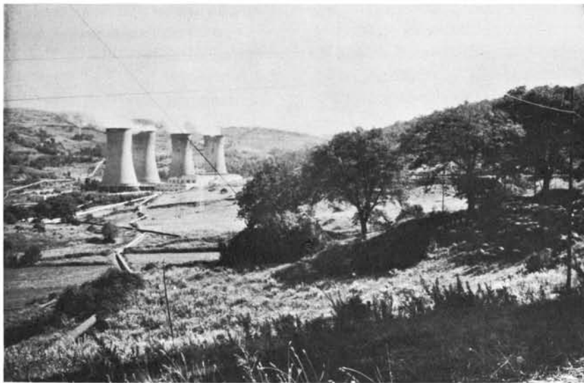
Figure 5. Larderello power plant with steam-gathering lines passing through an orchard in the foreground. This site has been used for electric power generation for over 60 years with only minimal environmental impact. (Photo by Ira E. Klein, U.S. Bureau of Reclamation)
