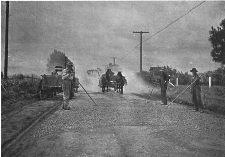
Macadam road under construction at Hood River about 1910.
