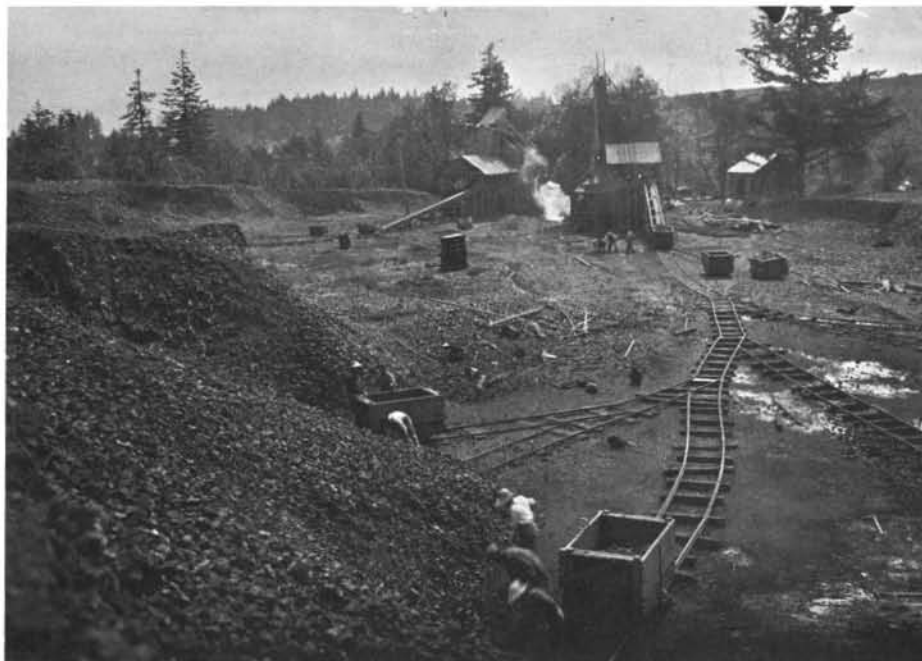
Ewald quarry, 2½ miles south of Salem in 1910. The dense hard, tough, and profusely fissured basalt was highly suitable for road rock.
