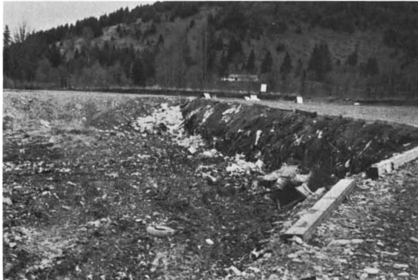
Lane County administers a clean appearing sanitary landfill at Cottage Grove. The Row River is within 100 yards of the left edge of the photograph and the refuse is buried at the level of the water table on the floodplain. No salvage is allowed.
