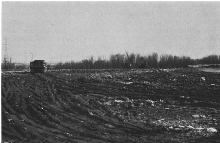
Soil layer being spread on refuse at the Swift Boulevard fill. Cover material is contracted from a nearby firm. A clay-silt is used in dry weather and a sandy loam for wet weather to improve workability.
