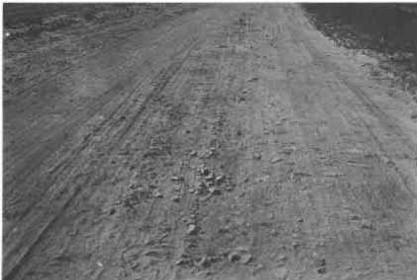
Macadam road at Pendleton about 1910; slightly ravelled surface was due to extremely dry weather.
