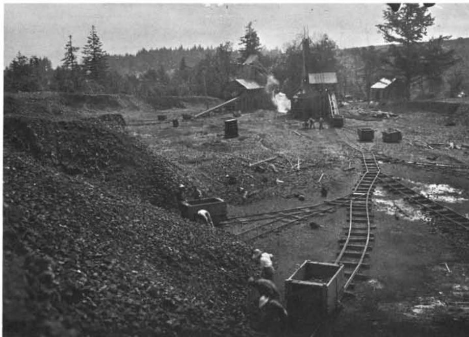
Ewald quarry, 2\frac{1}{2} miles south of Salem in 1910. The dense hard, tough, and profusely fissured basalt was highly suitable for road rock.
