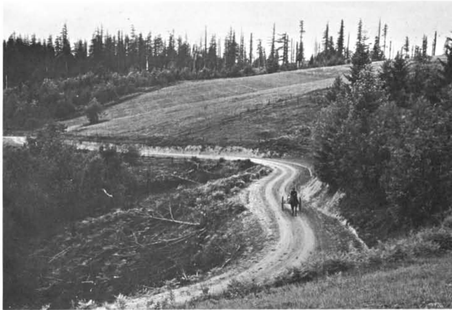
Germantown Road near Portland in 1910 showing proper location of a macadam road in hilly country.
