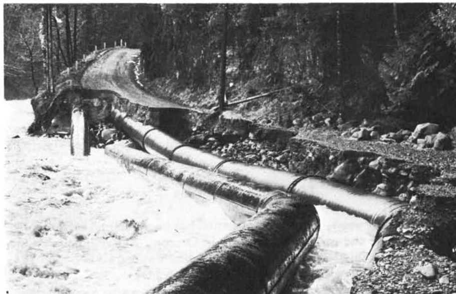
Figure 13. Stream-bank erosion on December 22, 1964 destroyed one conduit and threatened two others leading from Bull Run to Portland. Small-scale hazard damage concentrated in critical areas can result in catastrophe.
