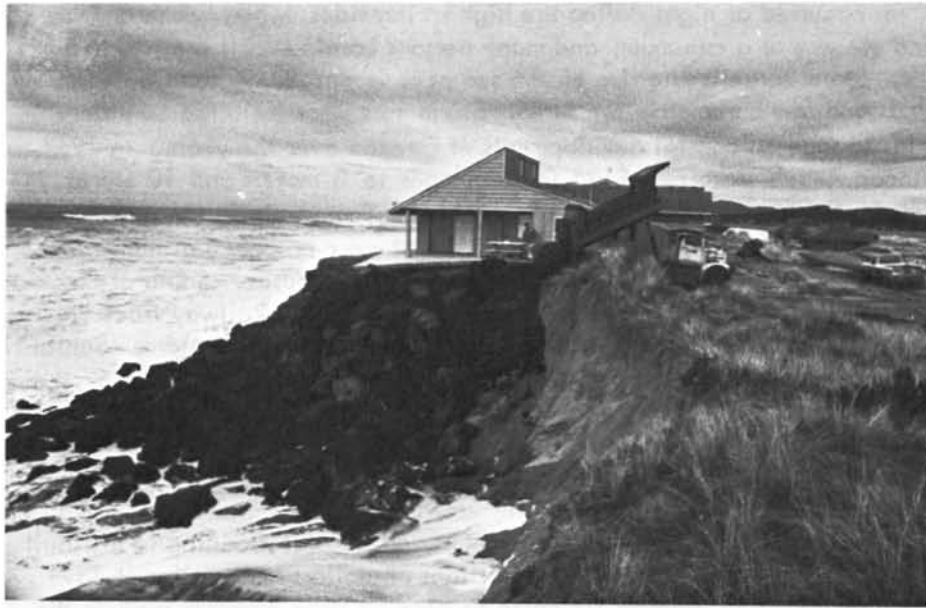
Figure 10. During the erosion of parts of Salishan Spit in the winter of 1973, riprap was placed around several houses to avert certain destruction. Sand spits are very sensitive to cyclic climatic activity and consequent changes in beach-zone sand budget.
