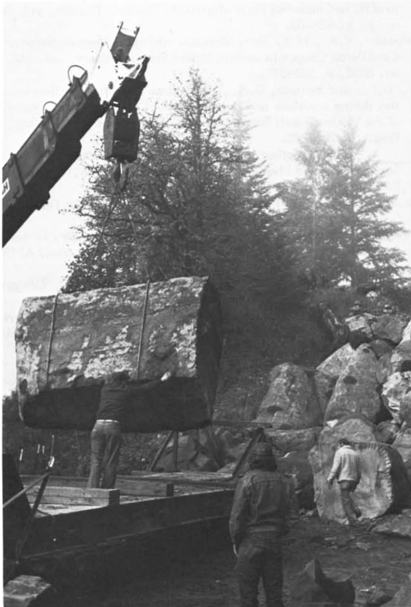
THE FIND - A 98-year-old Dilley resident and an article published in 1914 provided clues in the search for stone needed to repair fire damage at Pacific University's Marsh Hall. Here workmen load the giant block of sandstone, located at the old Boos Quarry, for shipment to Puyallup, Washington, where it was sawed and planed before being sent to the Forest Grove campus.
