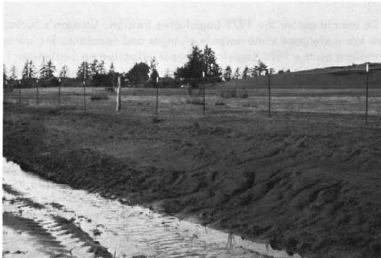
Same area as top photo. Pit has been leveled, top soil replaced, and grass seeded for pasture. Excavation is proceeding in foreground.
