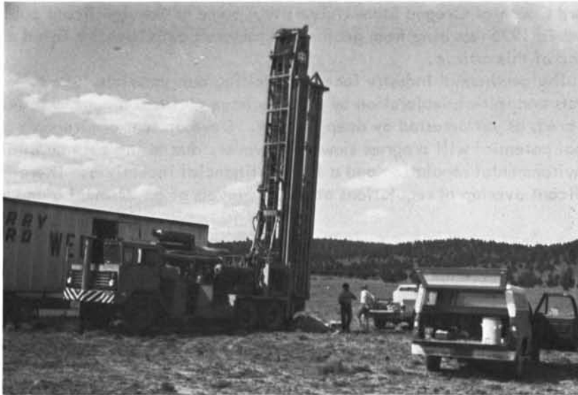
Department's geothermal-gradient test hole being drilled with a rotary air rig near the Brothers Fault Zone 17 miles west of Burns.
