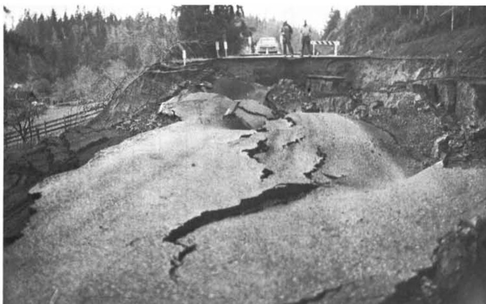
Figure 2. Slide along county road in Catching Slough Inlet, Coos County, during winter of 1974. Damage costs are difficult to determine from local and state highway maintenance records. (Photo courtesy The World , Coos Bay)
