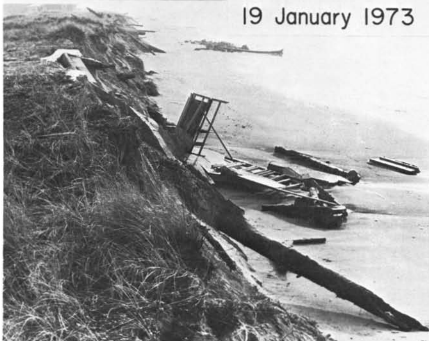
Figure 2. Erosion and destruction of the house under construction on lot 226 of Siletz Spit.
