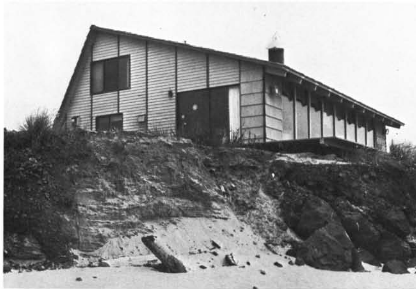
Figure 11. Erosion of the riprap fronting one of the homes, exposing some of the dune sands. Note small size of the rocks, which are easily removed by erosion.
