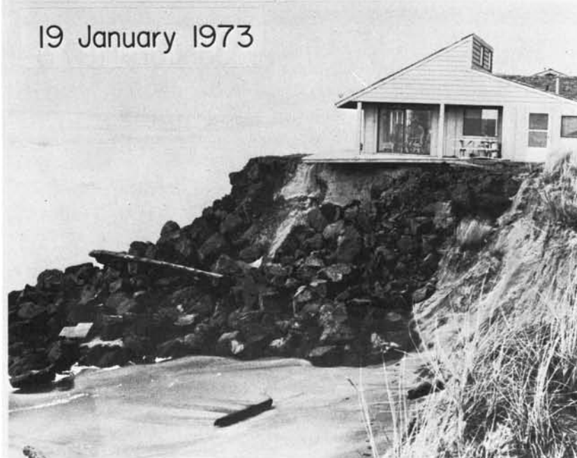
Figure 3. Erosion around the house on lot 229-A. Rapid erosion required placement of riprap fronting home in upper photo; but no riprap was installed in adjacent vacant lot, so erosion continued along the side as seen in lower photo.
