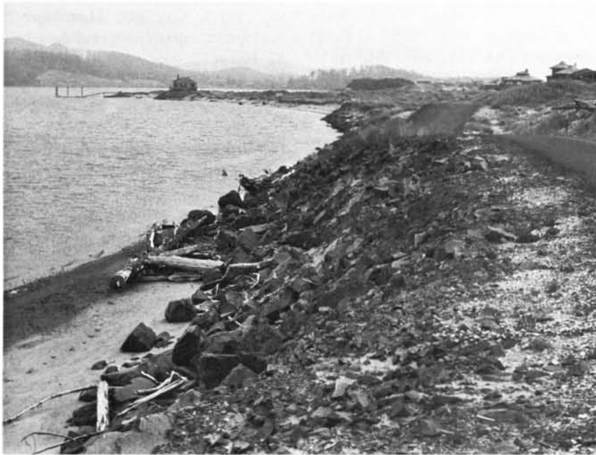
Figure 14. Riprap placed on the bay side of the spit to prevent or decrease erosion.
