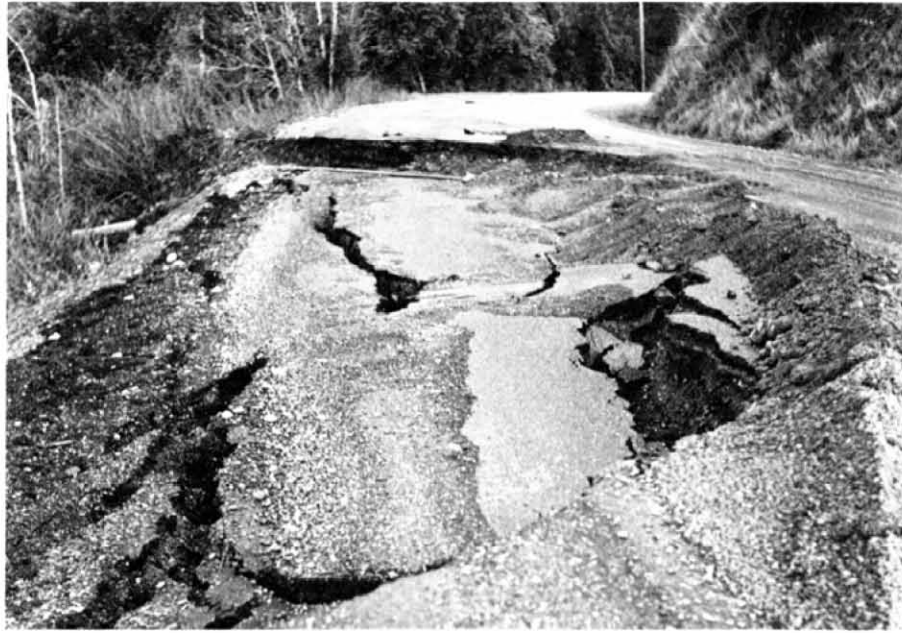
Slumping of roadway by undercutting of fill material is a common geologic hazard along western Oregon streams.
