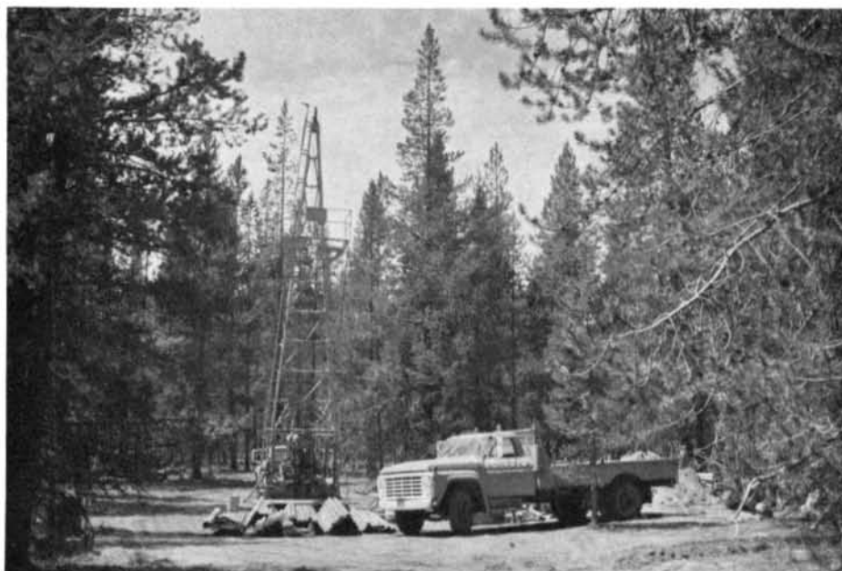
Figure 3. Thermal gradient drilling by USGS near Newberry Crater, July 1977.
