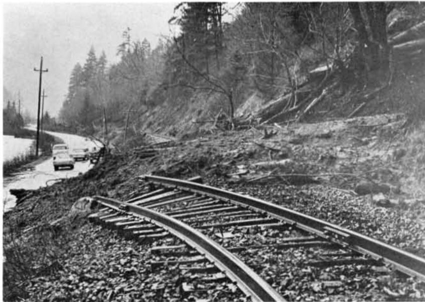
Figure 4. Debris flows emanating from steep terrain destroyed part of Union Pacific railway near Mapleton in winter of 1964-1965 (Schlicker and Deacon, 1974). (Photo courtesy Siuslaw News )
