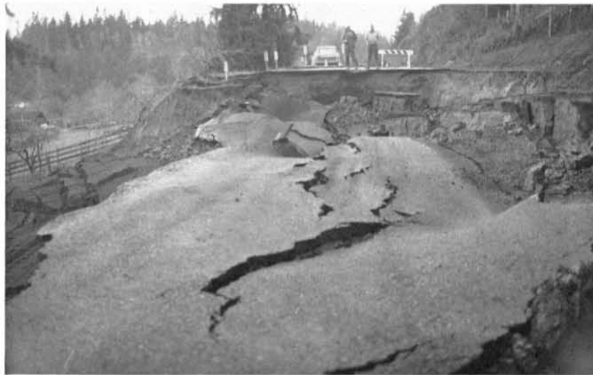
Figure 2. Slide at Catching Slough inlet in Coos County during 1974 flood is typical of damage inflicted on Oregon roads by geologic hazards (Beaulieu and Hughes, 1975). (Photo courtesy The World )
