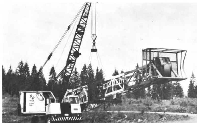
Derrick from Columbia County No. 1 being hoisted onto truck so it can be used in drilling Columbia County No. 4.
