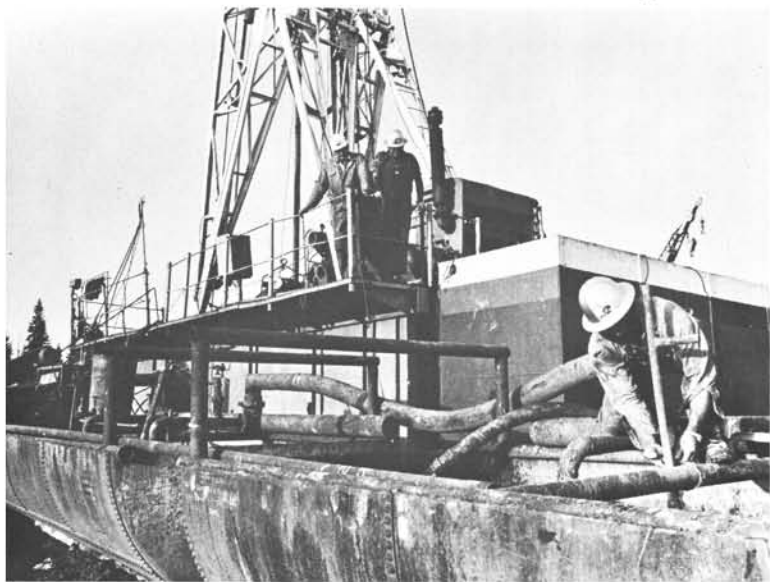
Checking mud tanks.
