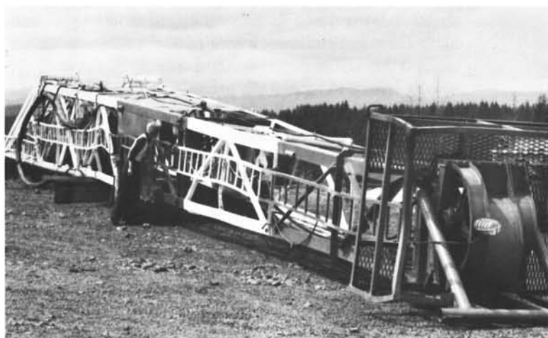
Derrick was lowered to ground after successful drilling of Columbia County No. 1 so it could be moved to next drilling site.
