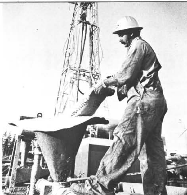
Adding "gel" to drilling mud.
