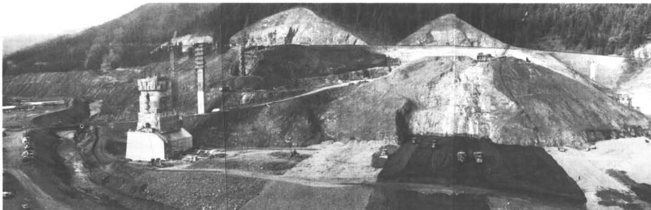
Figure 2. Panoramic view of one end of the U.S. Army Corps of Engineers Applegate Dam project, in which sand and gravel, Oregon's major mineral commodity, is being utilized as fill. When completed, the dam will be 242 ft high and 1,200 ft long and will contain 3 million cubic yards of fill. The tall concrete structure on the left is the intake tower for the dam. The downstream side of the dam is to the right.
