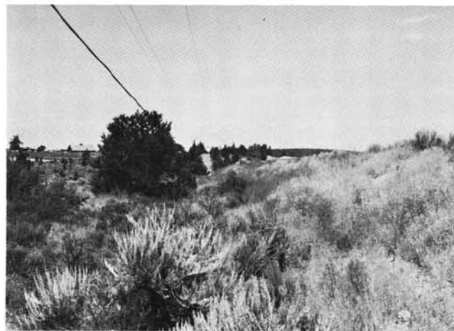
Leave strip and berm between road and pit at Cascade Pumice Company. The berm is made of stored topsoil overburden that can be respread as a seed base when mining is completed. In the meantime it provides a visual screen and sound barrier.
