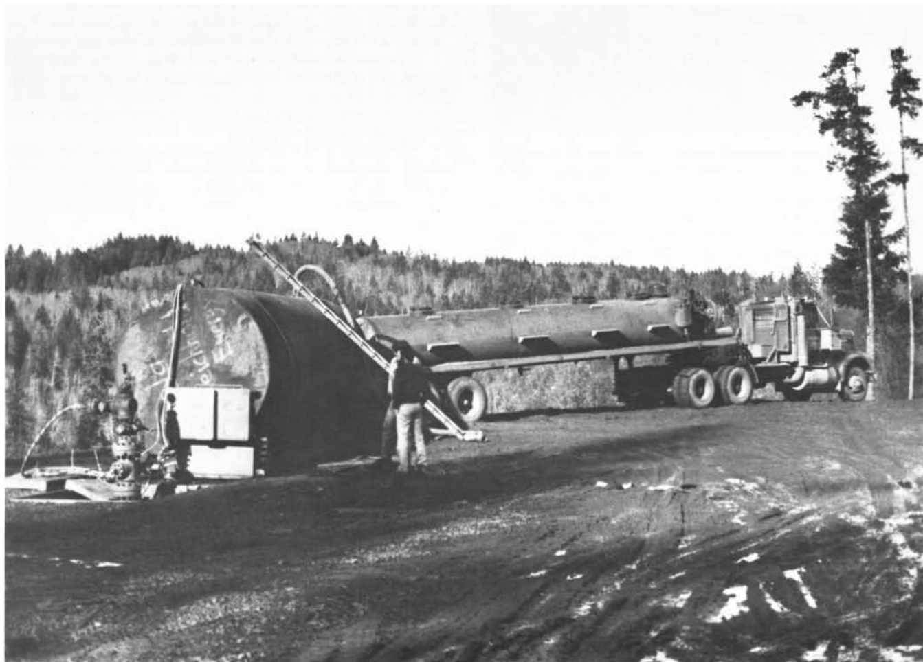
Reichhold Columbia County 13-1, Oregon's first salt-water disposal well. Vacuum truck in background is transferring salt water to holding tank for injection into the well.
