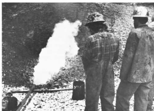
Flaring gas during initial potential test at Reichhold Columbia County 23-22, December 1983.
