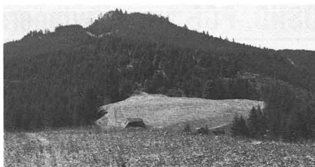
Oregon State Highway Division reclamation site on Rattlesnake Butte, a basalt quarry that yielded approximately 500,000 cu yd of rock. An area of 16 acres was reclaimed successfully. View is toward west. (MLR photo)
