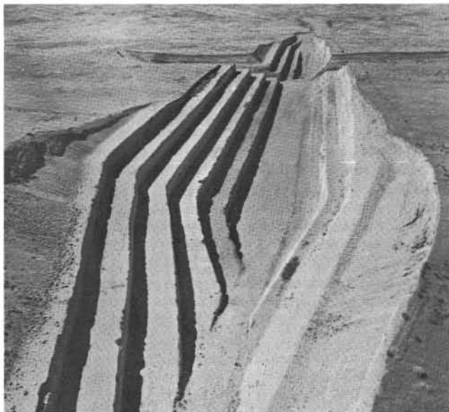
Exploratory excavation at PGE Pebble Springs nuclear reactor site. Two trenches with maximum dimensions of approximately \frac{1}{2} mi long, 400 ft wide, and 40 ft deep, before reclamation was begun. (Aerial photo courtesy PGE)
