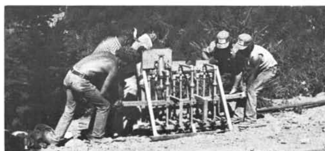
Moving blowout-preventer control manifold, Hutchins and Marrs Great Discovery 2, Douglas County, Oregon.
