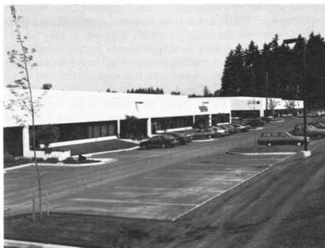
Commercial development on former part of Washington County basalt quarry. Area was backfilled with dry demolition waste, left to settle, sold, and developed. (MLR photo)
