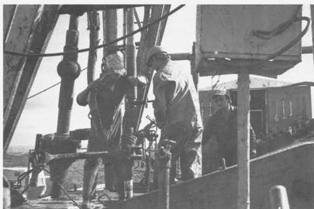
Driller and roughnecks running drill pipe into Columbia County 23-35, Mist Gas Field. The well was later plugged and abandoned.
