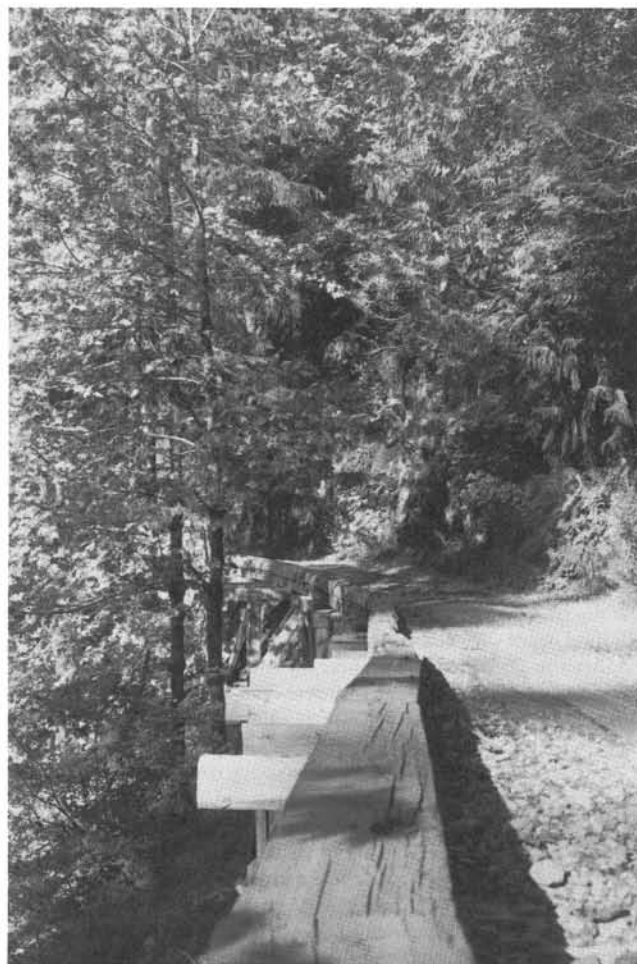
Stop 2. Half bridge, so called because the road is supported on one side by timbers and the other by the side of the valley, was required where the highly resistant rock of a large intrusion was encountered by the early miners in the North Santiam mining area.
