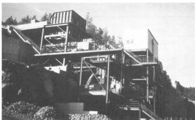
New wet-screening plant at Hanna Nickel Company high on the flanks of Nickel Mountain. Here, nickel-bearing, fine, weathered material is separated from unweathered rock and transported down the mountain as a slurry.
