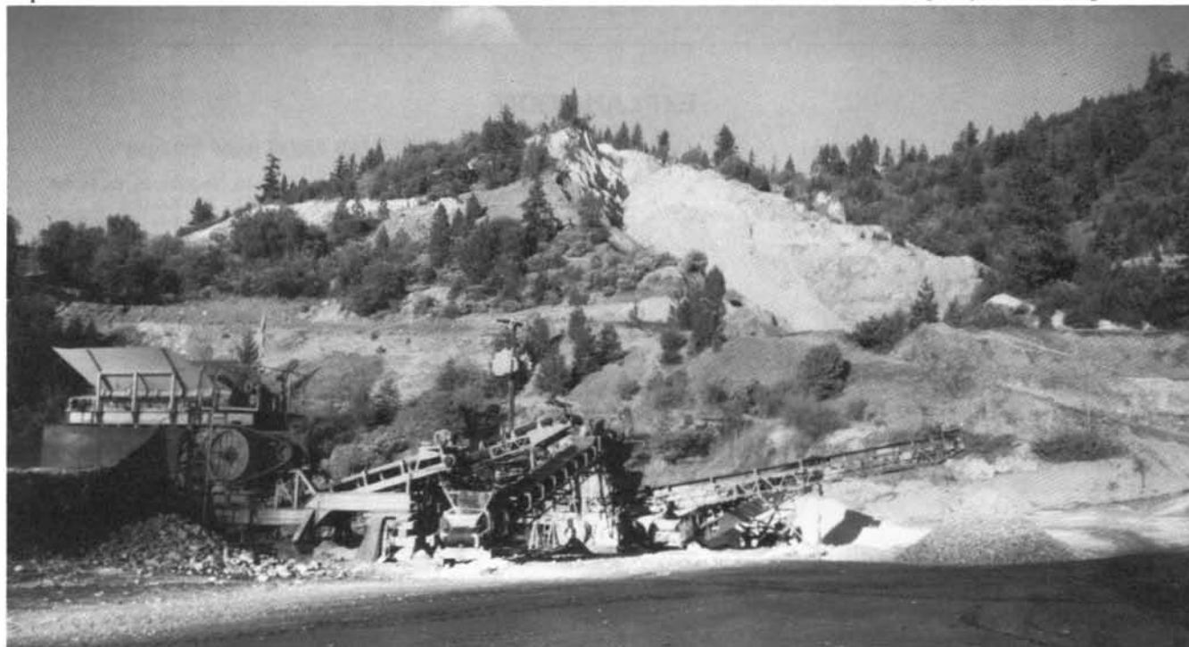
Bristol Silica and Limestone Company's mine in Jackson County. Open-pit quarry in background, crusher and screening plant in foreground. Here, silica rock used for decorative granules and silicon metal is produced.
