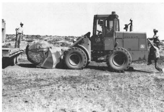
First attempts to load the boulder onto a truck were unsuccessful because the rock was too heavy. Note men trying to provide a counterweight at the back of the loader. Eventually the stone was pushed onto the truck.
