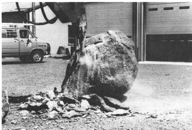
The boulder was eventually shaved to a smaller size by a hydraulic impact hammer mounted on an excavator.
