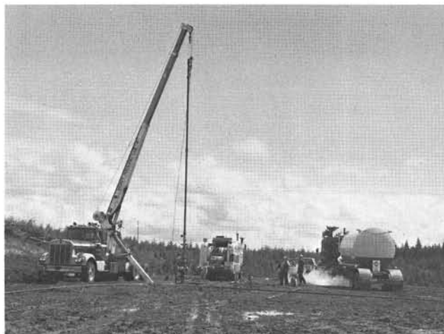
Preparations to flow-test the ARCO Longview Fibre 11-31-64 well.
