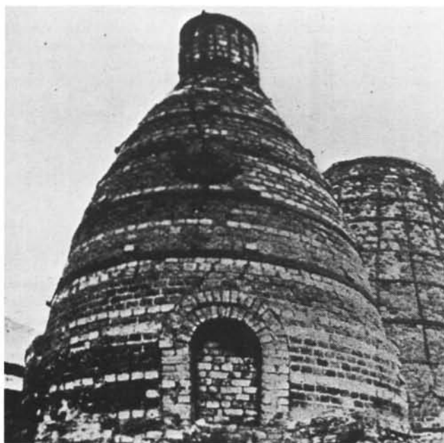
Figure 6. A bottle kiln for calcining limestone used in Aspdin's cement plant (around 1850). The kiln was 36 ft high, 17 ft in diameter at the base, and had a capacity of 21 tons of limestone per burn. It was much larger than Aspdin's original kiln, which had a capacity of about 6 tons of limestone. Early kilns of this type had a natural draft. Therefore, calcining and cooling might take several days, depending on the prevailing winds.
