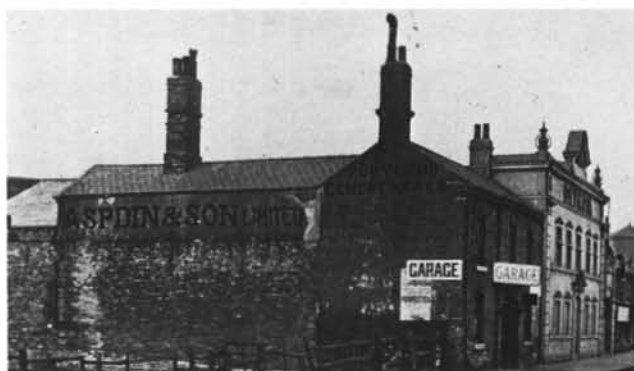
Figure 4. Aspdin's original cement plant in Wakefield, England, around 1860. The first extensive use of cement was in the Thames Tunnel in 1828. The engineer in charge of the project insisted on using portland cement and faced strong opposition because it cost more than twice as much as other natural cements then available. The cement proved worthy, and in the 1860's, nearly 70,000 tons of portland cement were used in the construction of the London sewer system. Aspdin's son William tried to keep his father's formula a secret by placing trays of copper sulfate in the kilns during the calcining process. The noticeable smell was intended to deceive competitors.
