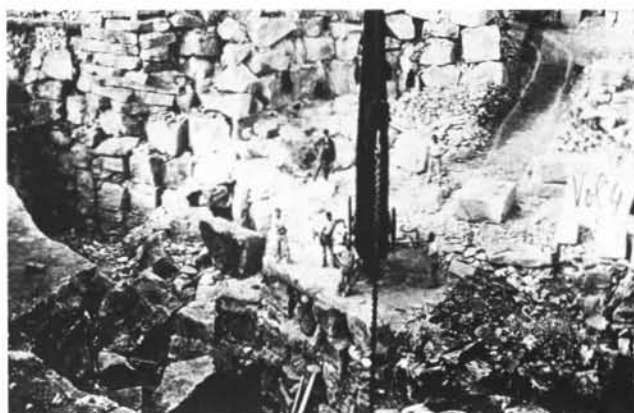
Figure 5. The famous limestone quarry on the Isle of Portland, south coast of England (around 1850). When Joseph Aspdin was experimenting with his cement concoctions, he had no efficient way of grinding the limestone. He found that the steel-rimmed wagons had sufficiently pulverized the limestone along the quarry road for his experiments. In 1825, while collecting crushed limestone samples along the main quarry road, he was arrested and fined for theft of public property.
