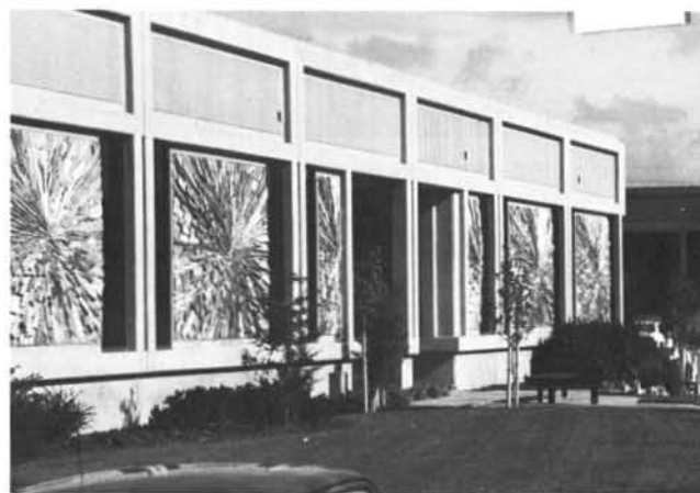
Figure 11. Tilt-up construction. The first tilt-up concrete buildings in the United States were used to store Army ammunition in the early 1900's. The thick, reinforced concrete walls are cast in place at the job site, allowed to harden, and tilted into place. Compared with other types, concrete tilt-up buildings take less time and money to construct and maintain. They require less insulation and cost less to heat in the winter and to cool in the summer compared with other types of buildings. They can be constructed quickly; some are completed 90 days from the time ground is broken. They eliminate the need of reinforcing beams and columns and require little long-term maintenance. Many innovative designs are used to make tilt-up buildings attractive. Photo by Don Dupras.
