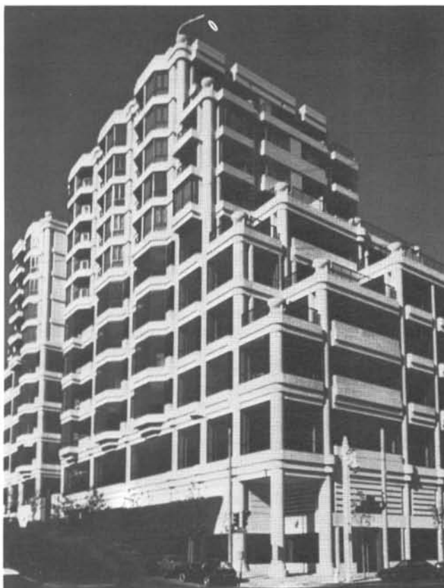
Ten-story building in San Francisco, California. Prestressed concrete panels were used on the exterior cladding because of their low weight, uniformity, and sharp profiles. Advances in concrete continue to expand its versatility. Photo courtesy of the Prestressed Concrete Institute.
