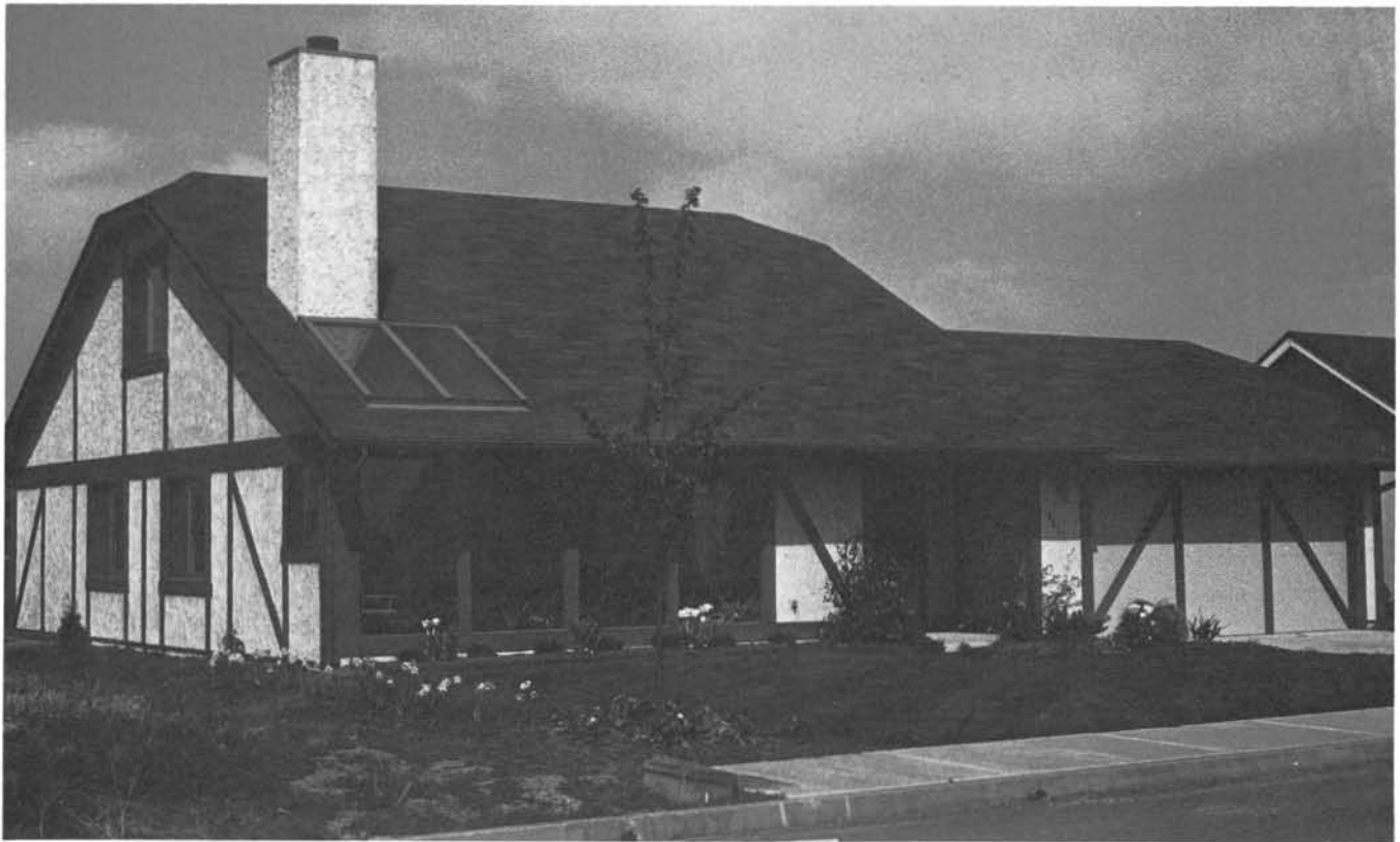
Award-winning private residence in Salem, Oregon, built with precast, lightweight, cellular concrete made of sand, cement, and foam. The new material allows easy handling, sawing, even nailing with regular nails. It also is rot- and termite-proof, resistant to fire, and has good sound-proofing and insulating qualities. This home also won an Oregon State Award based on energy efficiency, cost, and marketability. Photo courtesy of OCAPA.
