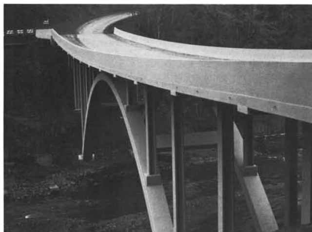
Fair Oaks Bridge at Sutherlin, Douglas County, Oregon, a structure that has received a number of awards for its use of concrete. The reinforced-concrete arch bridge uses both precast and cast-in-place concrete. Precasting of the arch ribs and columns saved greatly on forming costs, while the site-cast, post-tensioned deck system allowed the flexibility needed to construct grades and cross-slopes to meet traffic safety requirements. Photo courtesy of OBEC Consulting Engineers, Eugene, Oregon.
