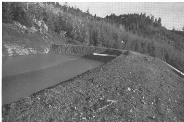
Bayview Transit settling pond with overflow system used to irrigate hillside vegetation.
