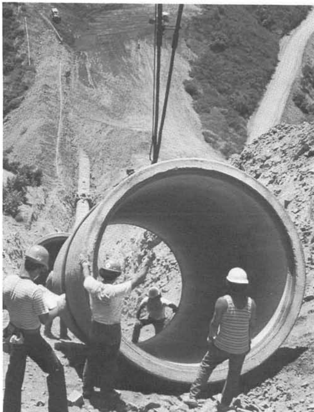
Construction of the San Diego, California, aqueduct in 1976. Each prestressed concrete-pipe section is 8 ft in diameter and weighs 40 tons. The aqueduct is being placed on a 55° slope near Fallbrook, California. Photo courtesy of Ameron.
