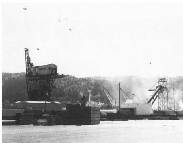
Hall-Buck Marine, Inc., bulk mineral loading facility at the Port of Portland Terminal 4. Soda ash from Wyoming is being transferred from unit train to freighter.
