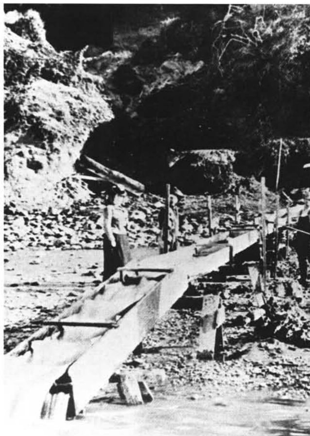
Mining the beach north of Newport with an 1890's "Long Tom" sluice box. Photo courtesy Lincoln County Historical Society.
