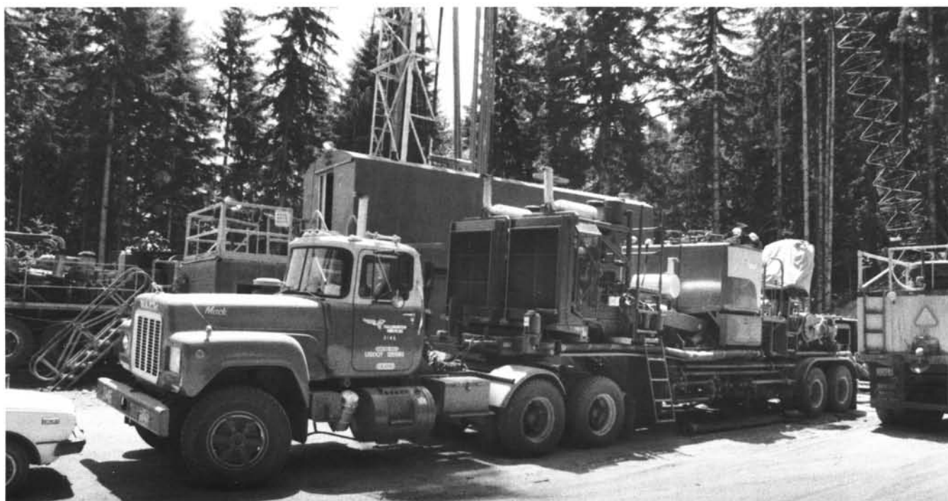
Figure 3. Cementing surface casing at the Nahama and Weagant Energy well CC 43-33-75, one of two successful gas producers drilled at Mist Gas Field during 1992. The surface casing consists of large-diameter pipe that is cemented in the well for the purpose of protecting fresh-water resources, anchoring blow-out prevention equipment, and maintaining the integrity of the surface hole. Truck pictured in foreground carries equipment to pump the cement down the hole.
