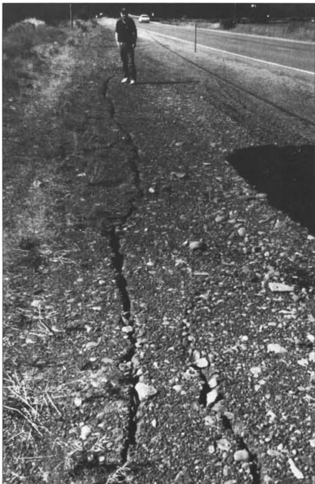
Figure 8. Linear cracks in the causeway fill south of Howard Bay bridge on Oregon Highway 140. These cracks were caused by slumping of fill in a westward direction, toward the right edge of the photograph.
