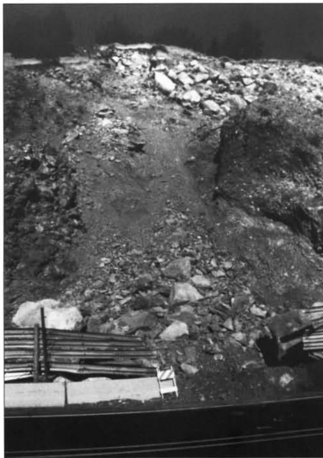
Figure 6. Rock slide from Modoc Rim, 2.9 km (1.8 mi) south of the town of Modoc Point and adjacent to U.S. Highway 97 (Locality 3, Figure 2). Note breach in roadside barrier and impact marks in highway pavement caused by large boulder that hit southbound vehicle and came to rest on road. The boulder was pushed off the road before the photograph was taken and is visible just behind the right side of the breach.
