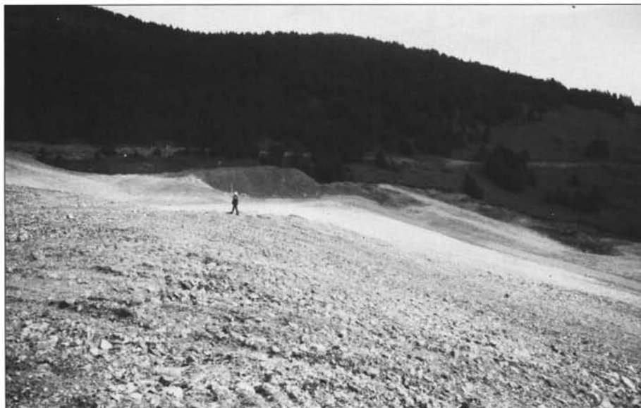
Figure 2. Waste dumps at Homestake's Nickel Plate Mine in British Columbia is being reshaped to relatively flat (3:1) slopes, which are much more successful in revegetation efforts than steeper slopes.
